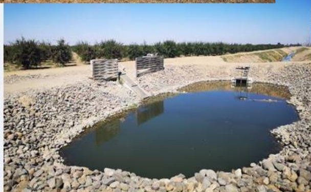
Grasslands Bypass Project, Central Valley CA Engineered system for collecting all contaminated drainage water from 97,000 acres of high value farmland, protecting a significant complex of wetland habitats in the San Joaquin River. Drainage water is used to grow salt tolerant wheatgrass (top right) on 6,000 acres of marginal land, used as a fodder crop for nearby dairy farms.
