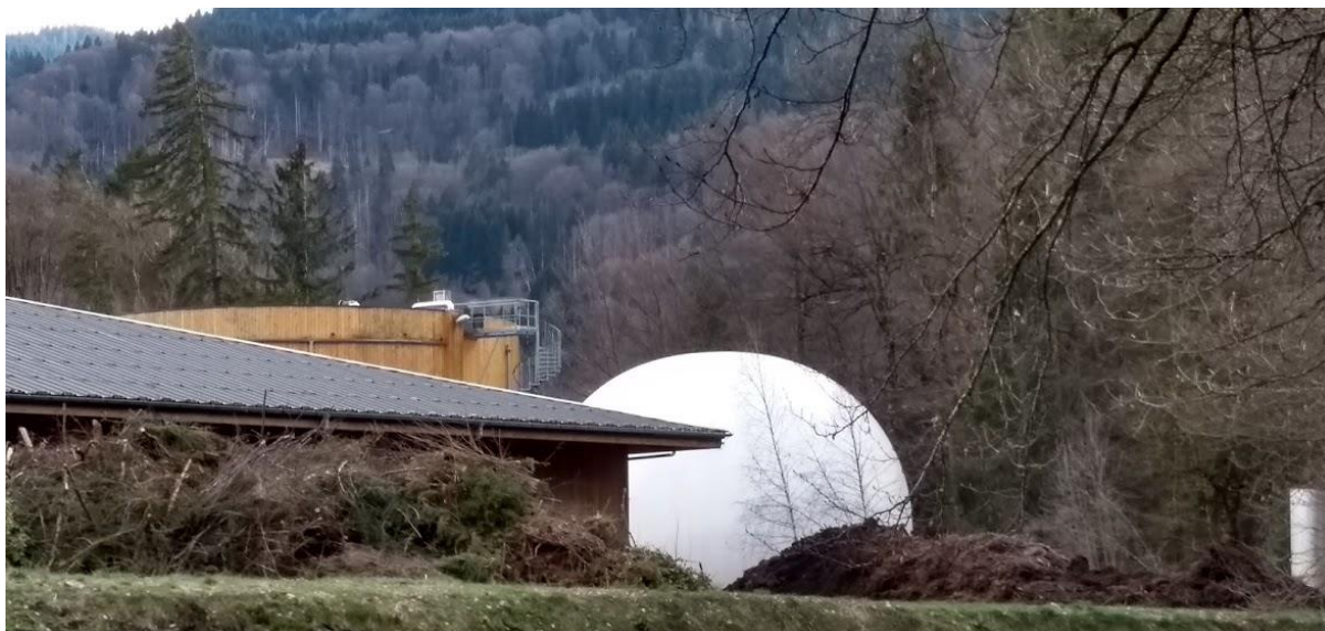
Figure 16. French biogas plant visited fed on food waste collected from numerous commercial establishments. Waste that was not readily fermentable was treated by windrow composting
