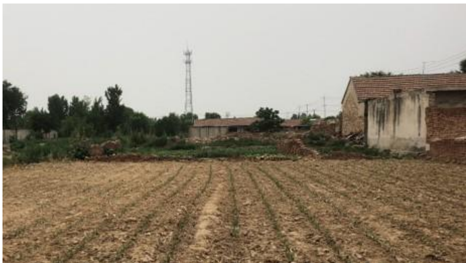
Figure 10 China land consolidation. A rural village in transition - undergoing demolition (Source: Author)
