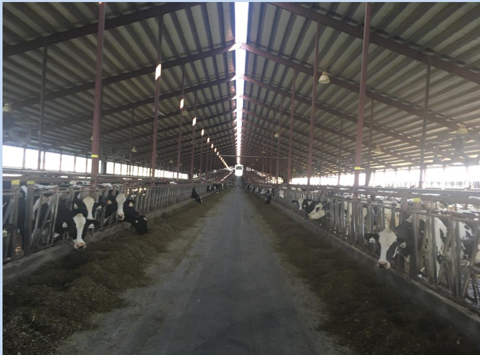
Figure 15: One of 4 cubicle barns at Lake Breese
