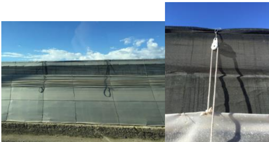
Figure 14: (Left) Pulley system used in Almeria and (right) side vents with pulleys
