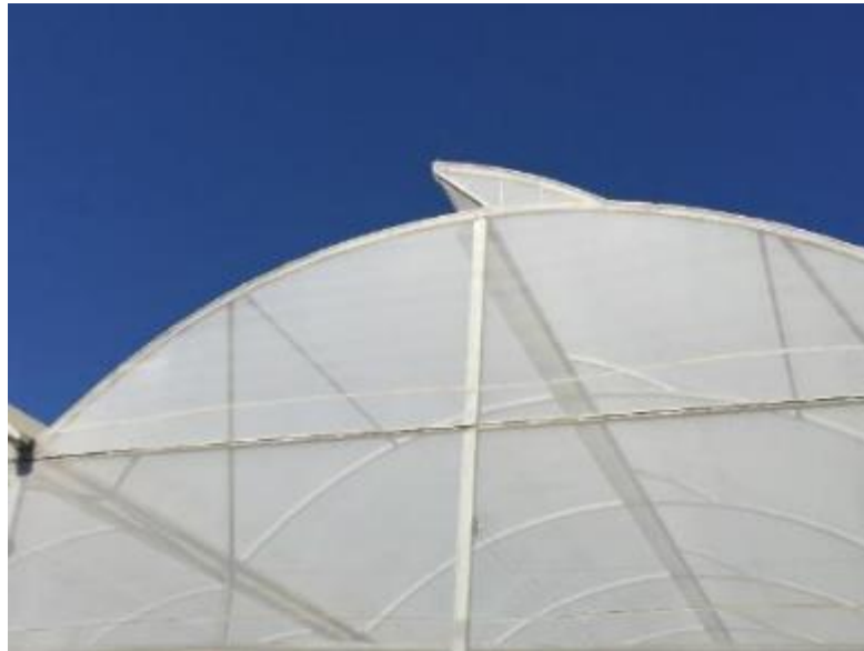
Figure 4: Example of top vent similar to permanent saw tooth vents in Brazil (Author)
