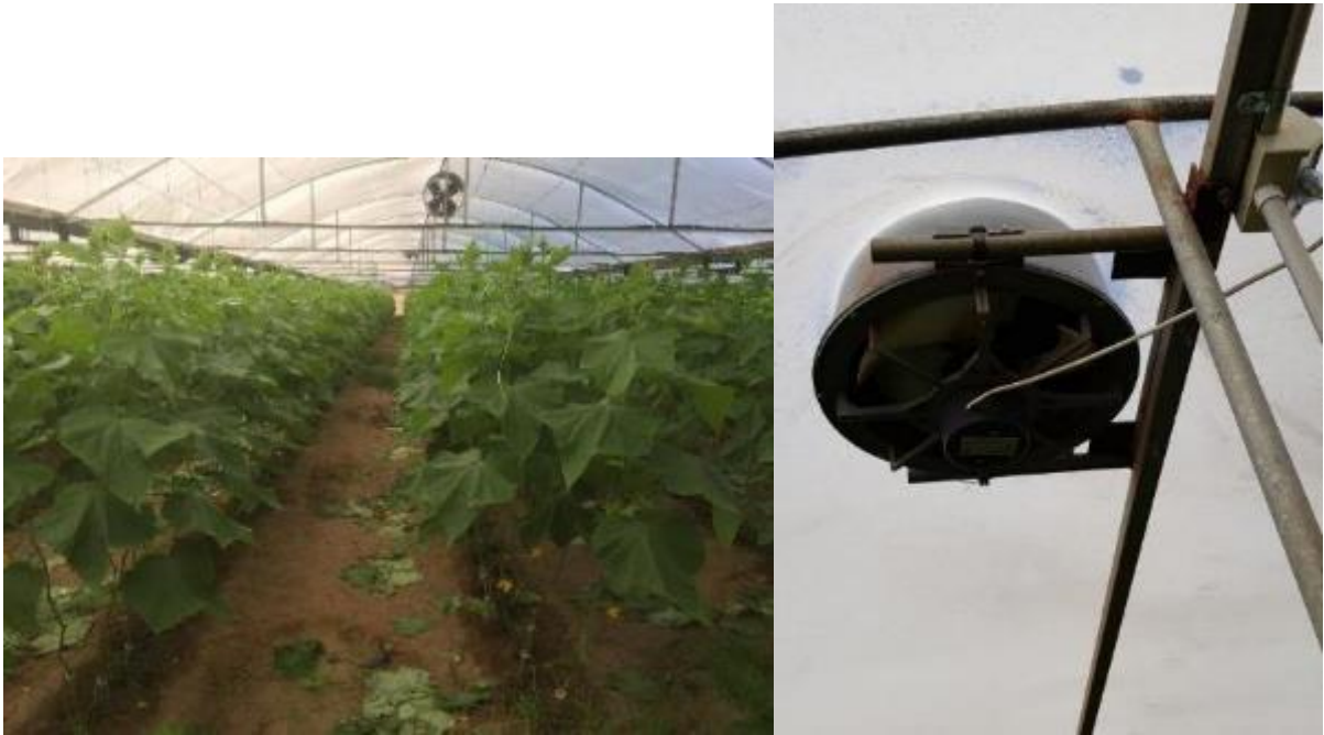
Figure 11: Fans in the roof to extract heat and humidity currently being trialled at Sun City Produce, Geraldton (Author)
