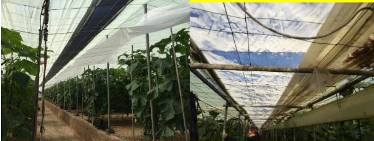
Figure 8: Small flat vents in Spain (Author)
