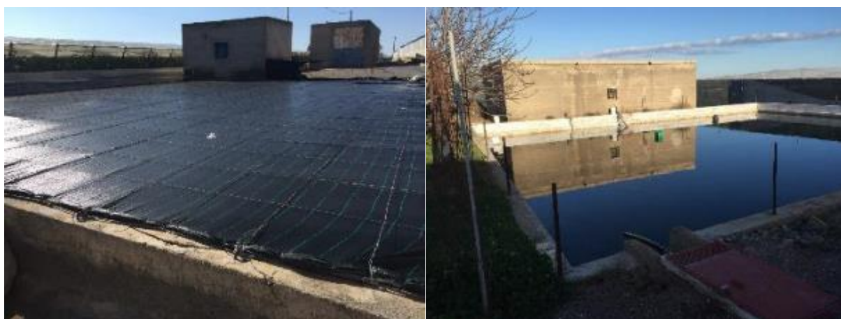
Figure 24: Water Storage, Almeria, Spain (Author)
