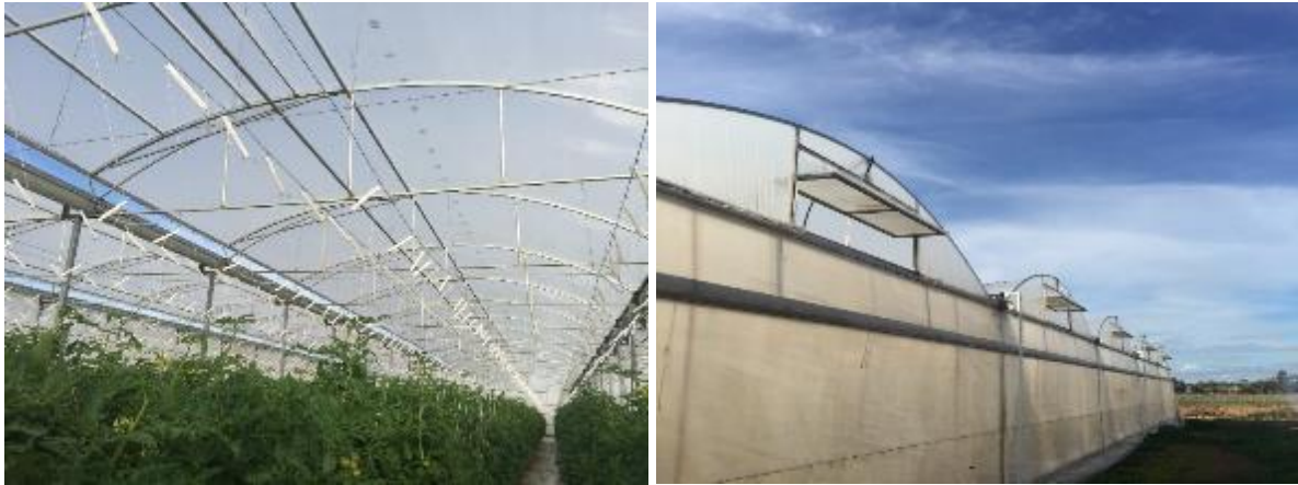
Figure 6: Roof and window vents, Adelaide 2018 (Author)
