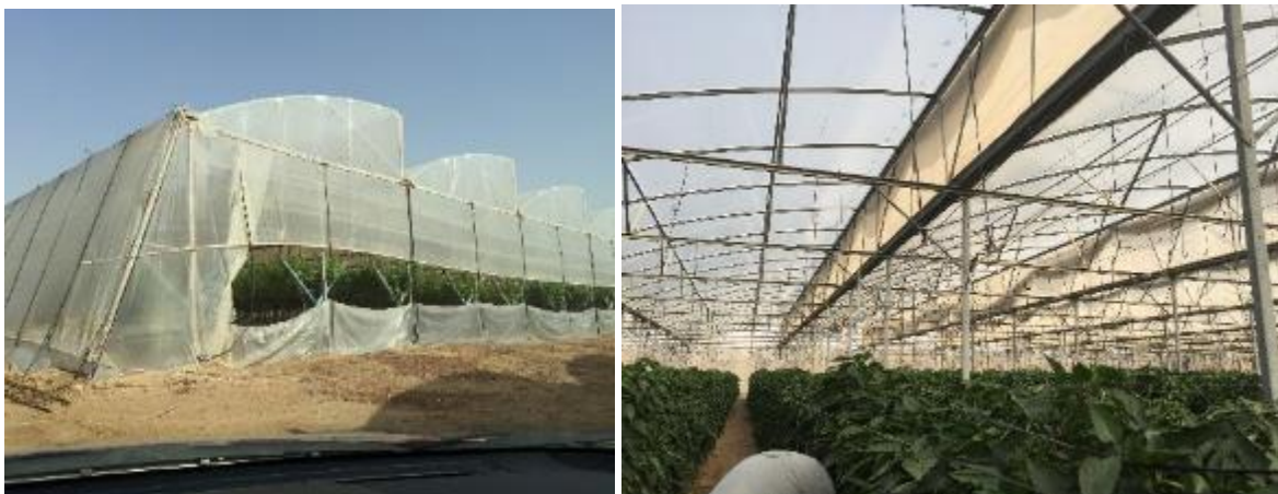
Figure 3: Greenhouses with permanent sawtooth vents (Author)
