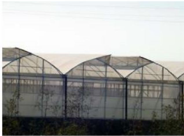
Figure 9: Gothic-type multi-span greenhouse with windows in the ridge (Martinez et al, 2016)
