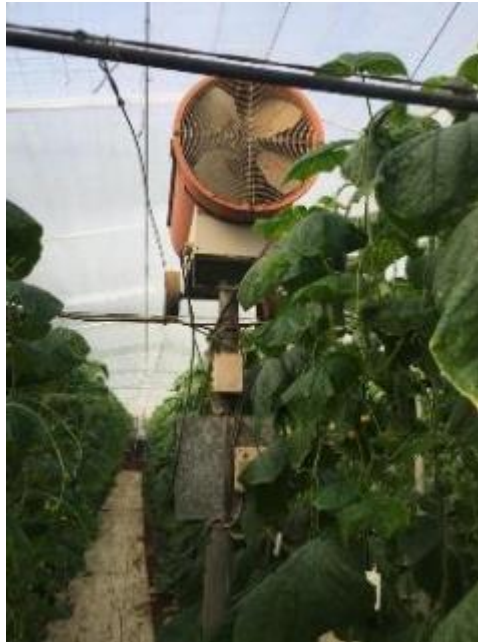
Figure 17: Gas and diesel heaters (Author)
