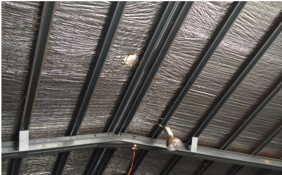
Figure 6: Roof insulation to keep workers cool
