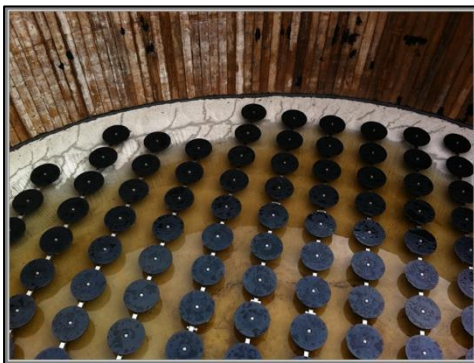
Figure 3: Nitrification – compressed air is blown through the liquid. This process converts the ammonia or ammonium to nitrite.
