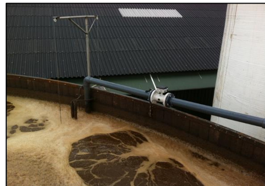
Figure 3: Denitrification – results in the reduction of the nitrates to nitrogen gas.
