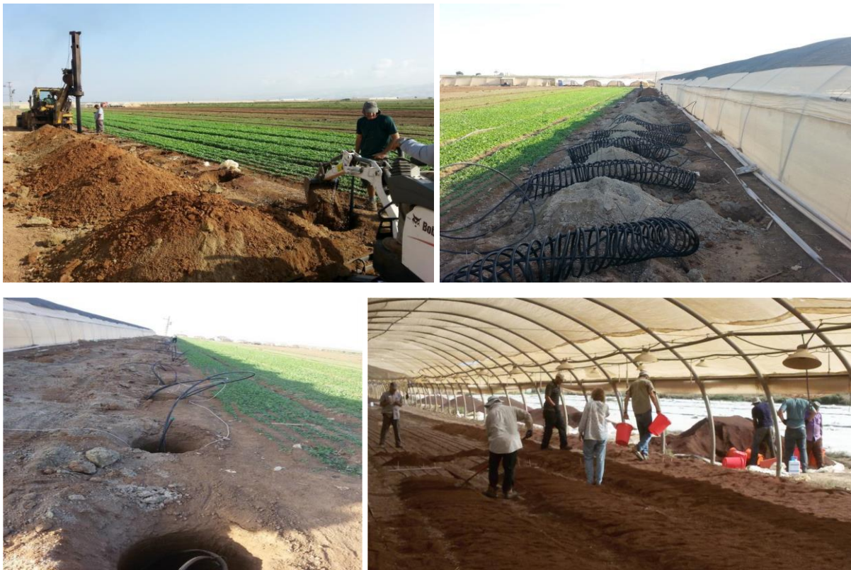
Figure 4: ROOTS being installed at Jordan Valley Herbs, Israel (clockwise from top left) digging and installing GSHE coils for root zone heating and cooling; coil ready to be installed in pits; covering the root zone growing area; coils installed in pits (Photos courtesy RootsSAT) Jordan Valley Herbs
