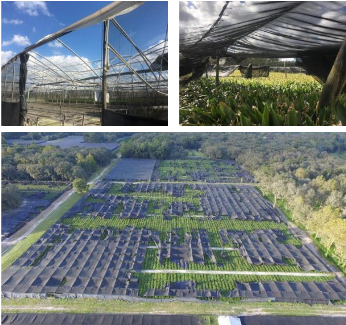
Figure 7: Damage from strong winds during tornado event north of Florida (23, January 2017) Costa Farms, South Florida; major structural damage at Ronald Harris Ferneries following Hurricane Matthew; and Albin Hagstrom and Sons, causing millions of dollars of damage to shadehouses in Central Florida, August (2016) (bottom photo courtesy Albin Hagstrom and Sons).
