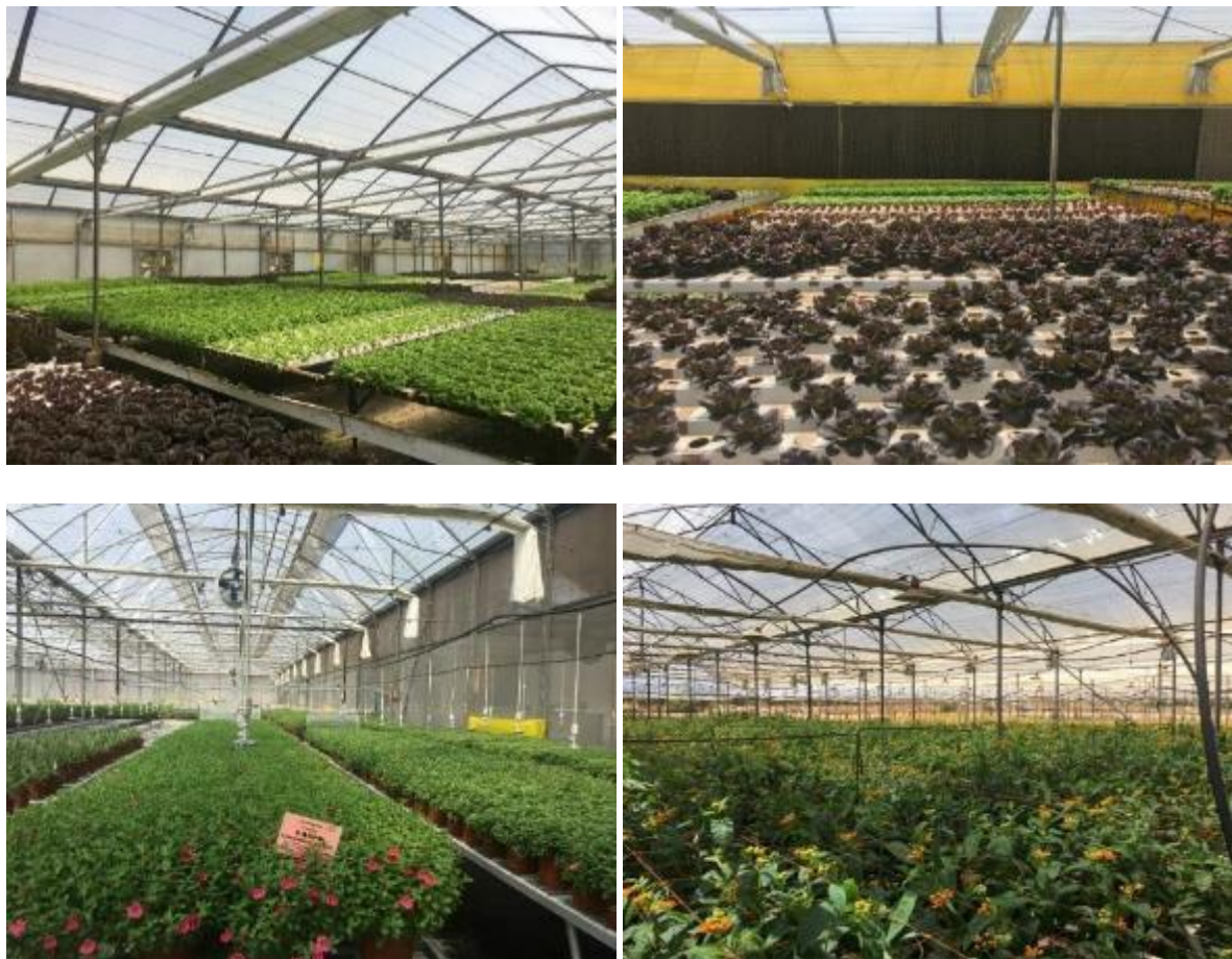
Figure 3: Controlling the microclimate in protected cropping facilities in subtropical climates (clockwise from top left) extraction fans; and cooling pads installed in medium-tech greenhouse for hydroponic lettuce production (Mavor Hydroponic Lettuce, Israel); butterfly vents, retractable thermal screens and circulation fans in vegetative cutting production facility, TicoPlant, Costa Rica; retractable screens and HPS lamps for increased day length (Gafni Farms, Israel)
