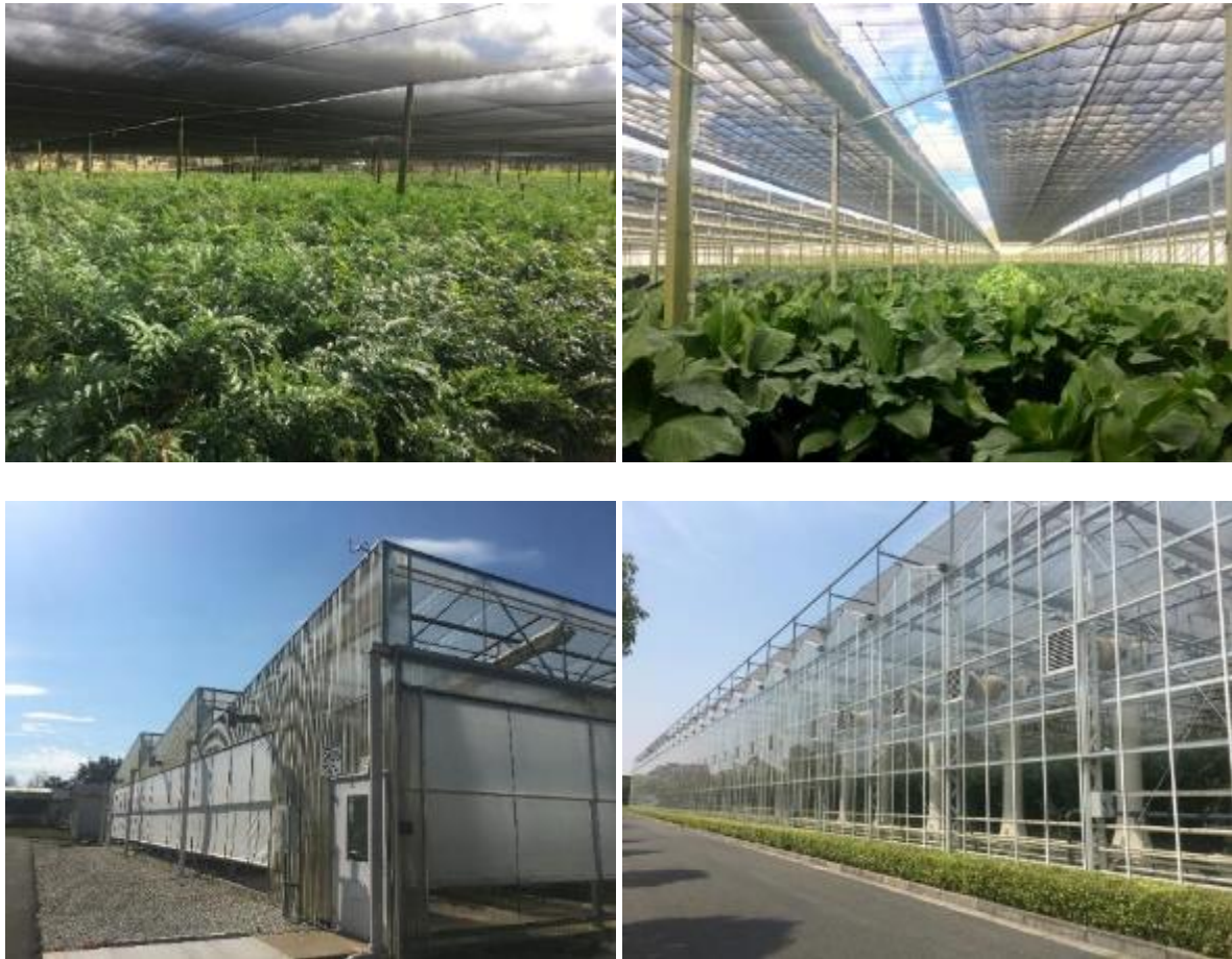
Figure 2: Variety of protected cropping structures (clockwise from top left) low-tech timber and cable shade house (73% shade), Ronald Harris, Florida; Cravo retractable roof greenhouse, Butler's Foliage, Florida; medium-tech, semi-closed polycarbonate, saw-tooth design greenhouse, Gainesville, University of Florida; high-tech glasshouse Dushi-green, China.
