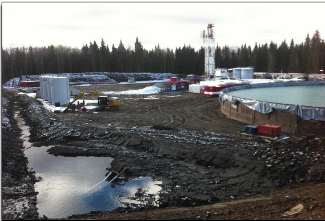
Figure 13. Tamarack Drilling Site, 2016. Fracking supply water holding tank right, intercepted water supply foreground left, with pump in it. (Source: Author).
