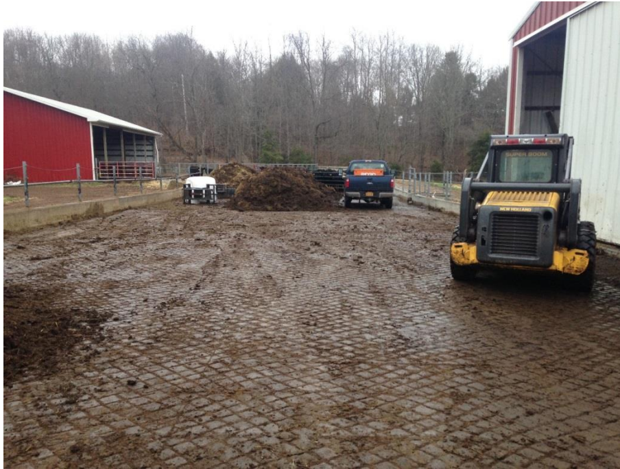
Figure 17: Livestock collection yard in New York State to prevent poaching and manure runoff
