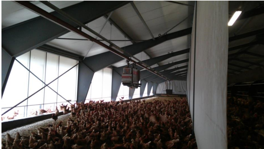
Figure 19: Forage feeding system by JH Staldservice A/S in operation, Jutland, Denmark
