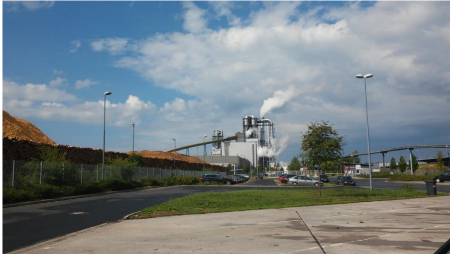
Figure 45: Finding heat sources for insects. This giant timber processing Fibreboard plant in Germany supplies surplus recovered heat from their process to the insect rearing houses at Hermetia AG.
