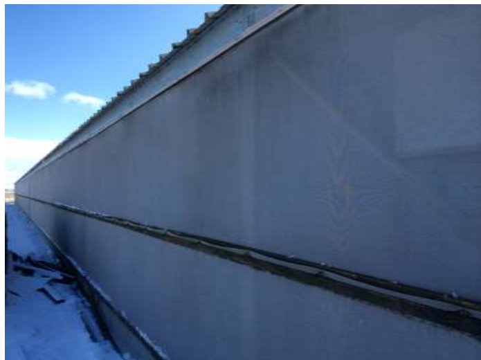
Figure 12: Shed with side inlets which are covered year round to exclude flies
