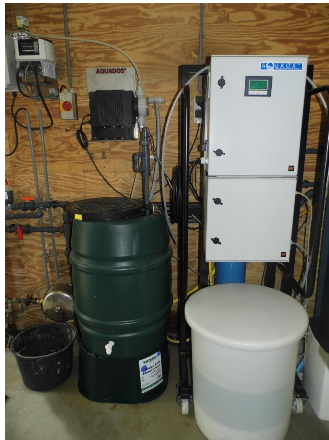
Figure 5. Image showing the Aquaiox machine supplying electrolysed water on a broiler farm in Holland
