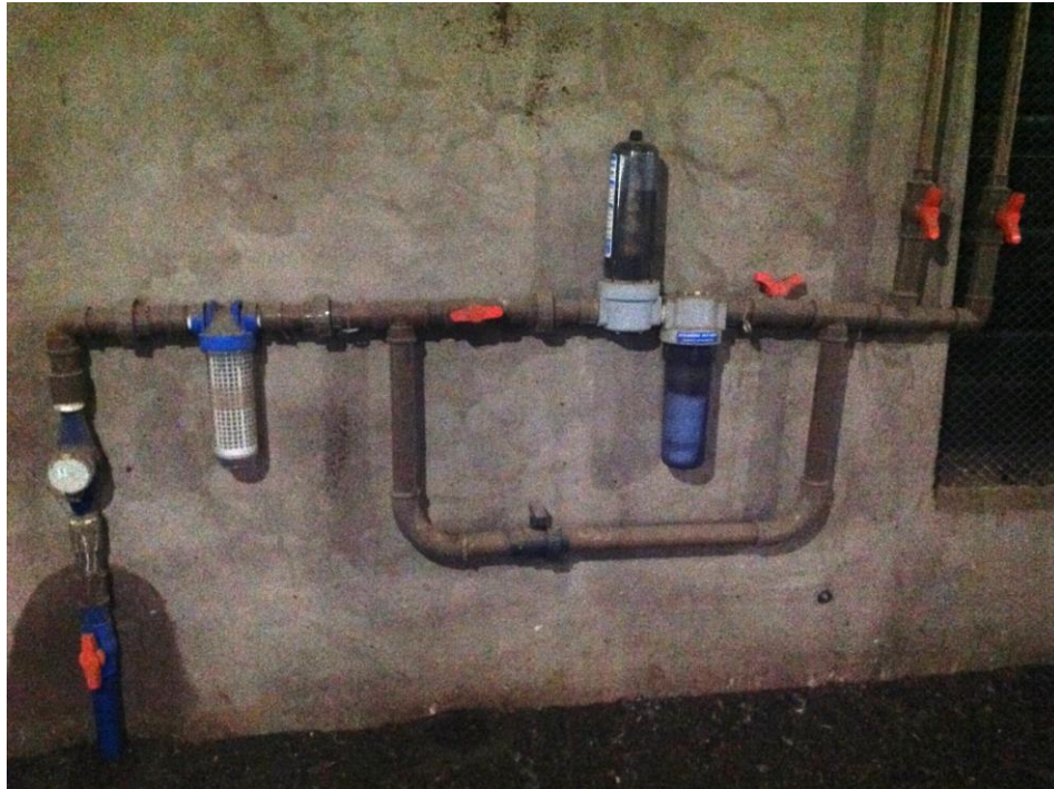
Figure 4. Image demonstrating the simple system used on Brazilian farms to administer chlorine as a water sanitizer. The two containers on the right of the picture are both adding products to the water - chlorine via one and a product to reduce condensation on the pipes in another.
