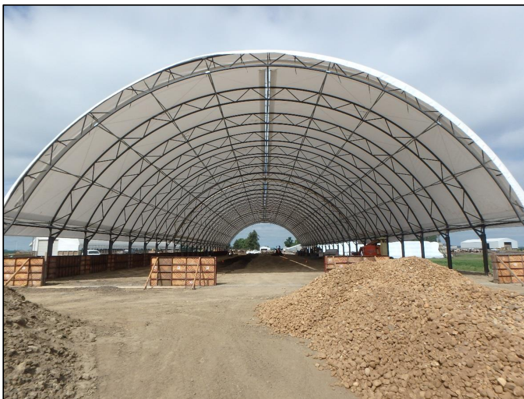
Figure 58: New 1,000 head finishing hoop being built in Minnesota as part of a 5,000-head all-dairy steer unit
