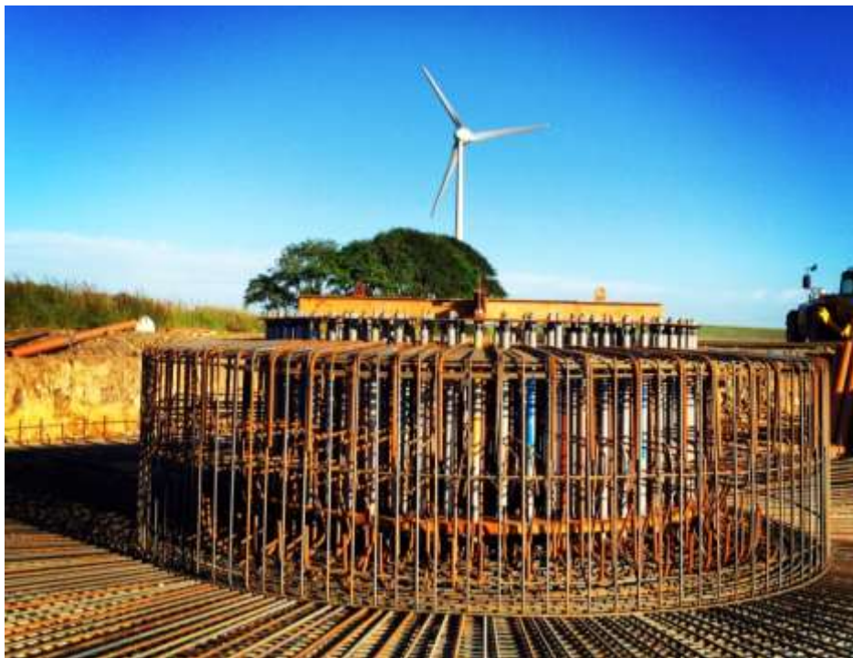
Figure 19: The foundation steel rebar of the next turbine at Inverquhomery, my family farm.
