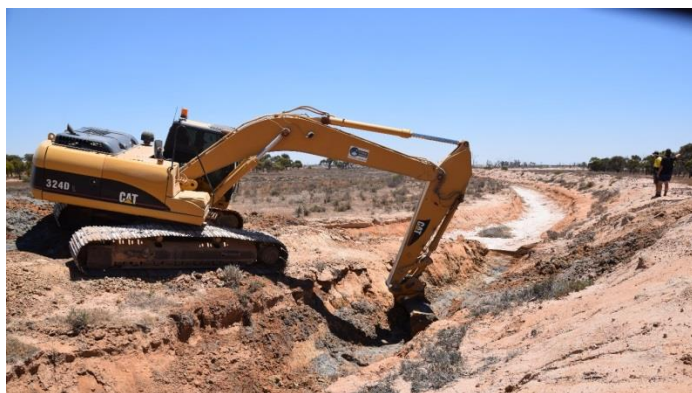
Figure 18. Excavator clearing drainage canals for saline ground water in Western Australia
