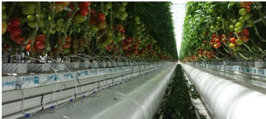
Figure 2 Air tubes under the gutter in The First Faber HYBRID X GH built in South Australia featuring a gutter height of 7.3 meters, diffused glass and a white powder coated construction. Royal Brinkman supplied and installed the complete computer (Priva), electric and irrigation System (Source: www.fabergreenhouses.com.au )
