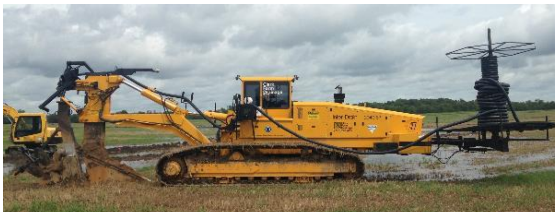
Figure 11: Inter-Drain trenchless plough.
