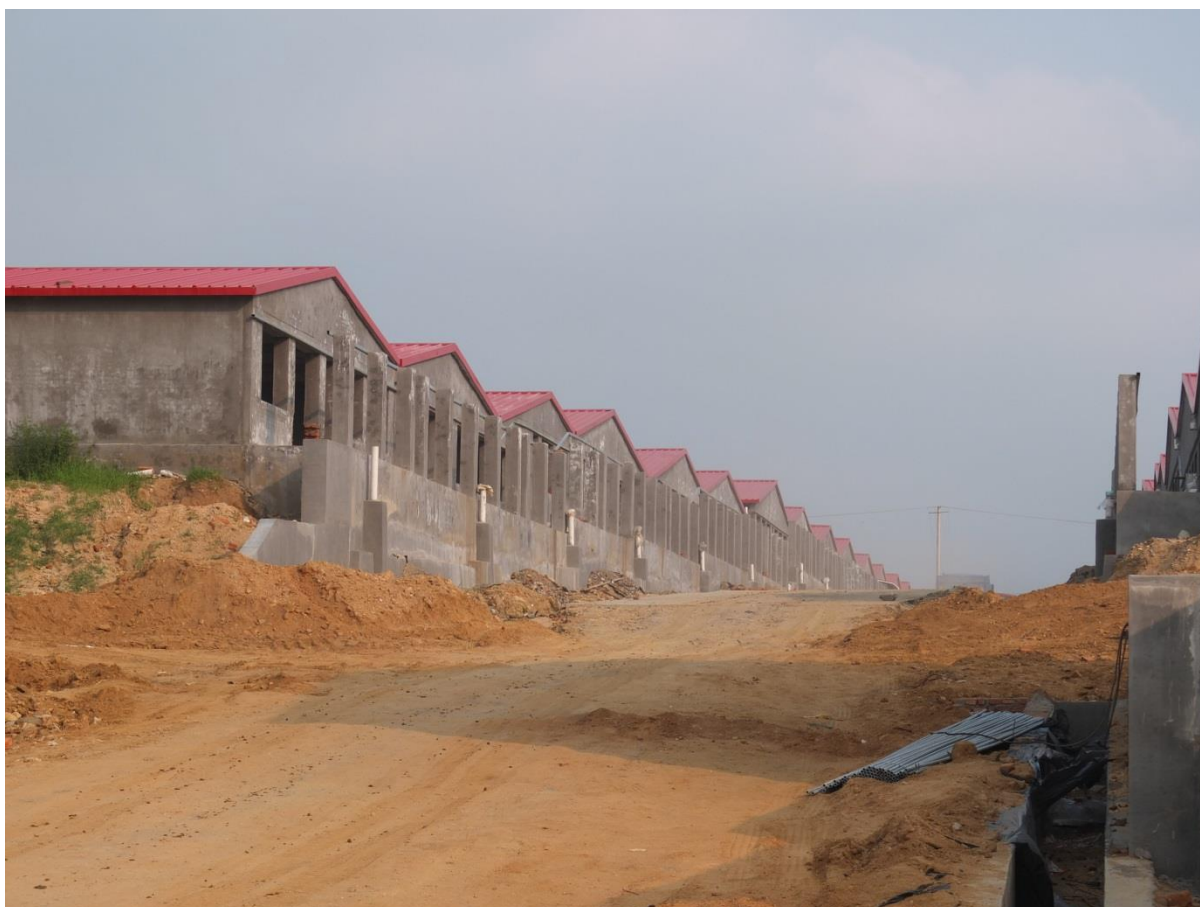
Picture 3 : finisher buildings under construction in Shangdong Province, China – the scale and speed of growth in China is fascinating.
