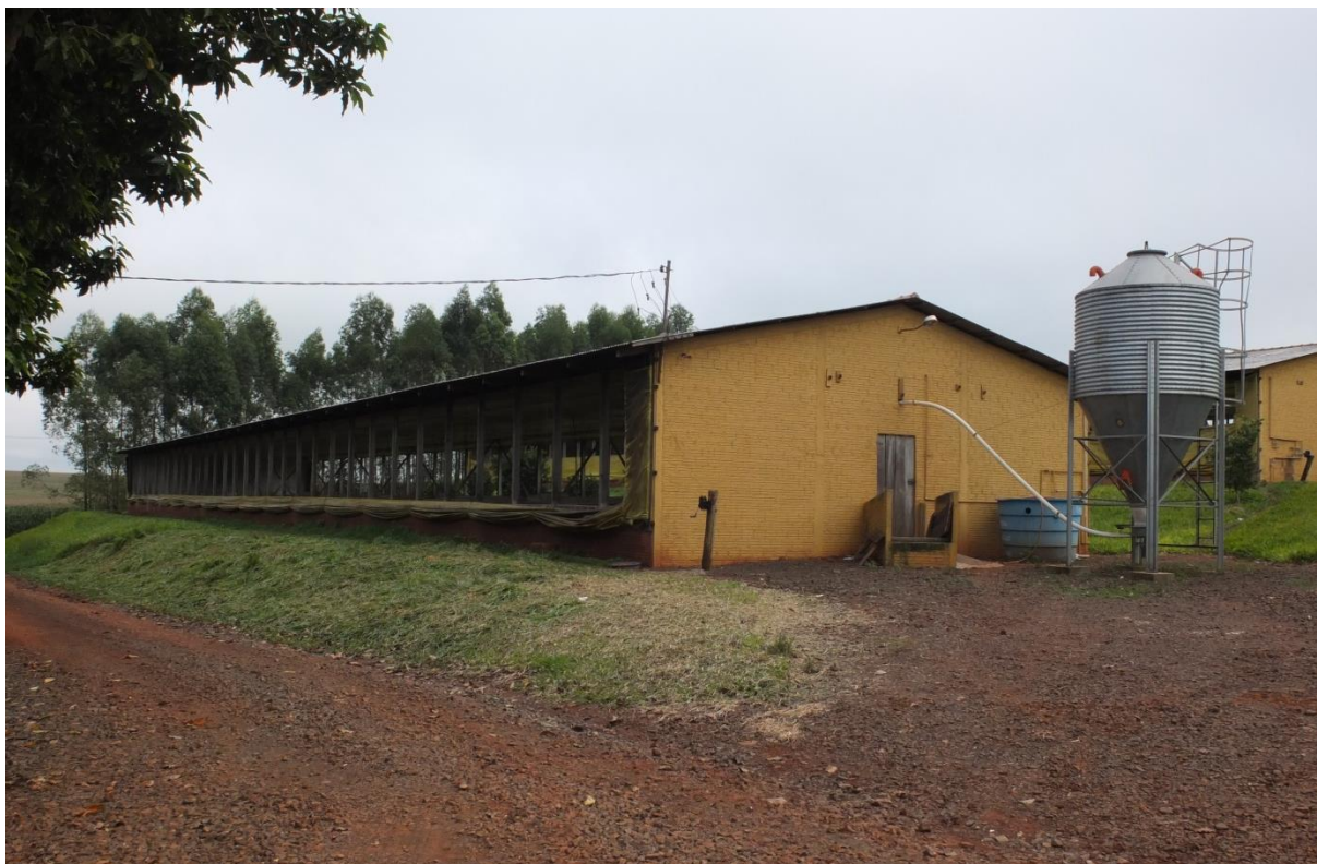
Picture 4 : typical finishing pig buildings in Parana state, Brazil. These solid floor buildings are washed down daily by hand as the slurry is used in an anaerobic digestion plant.
