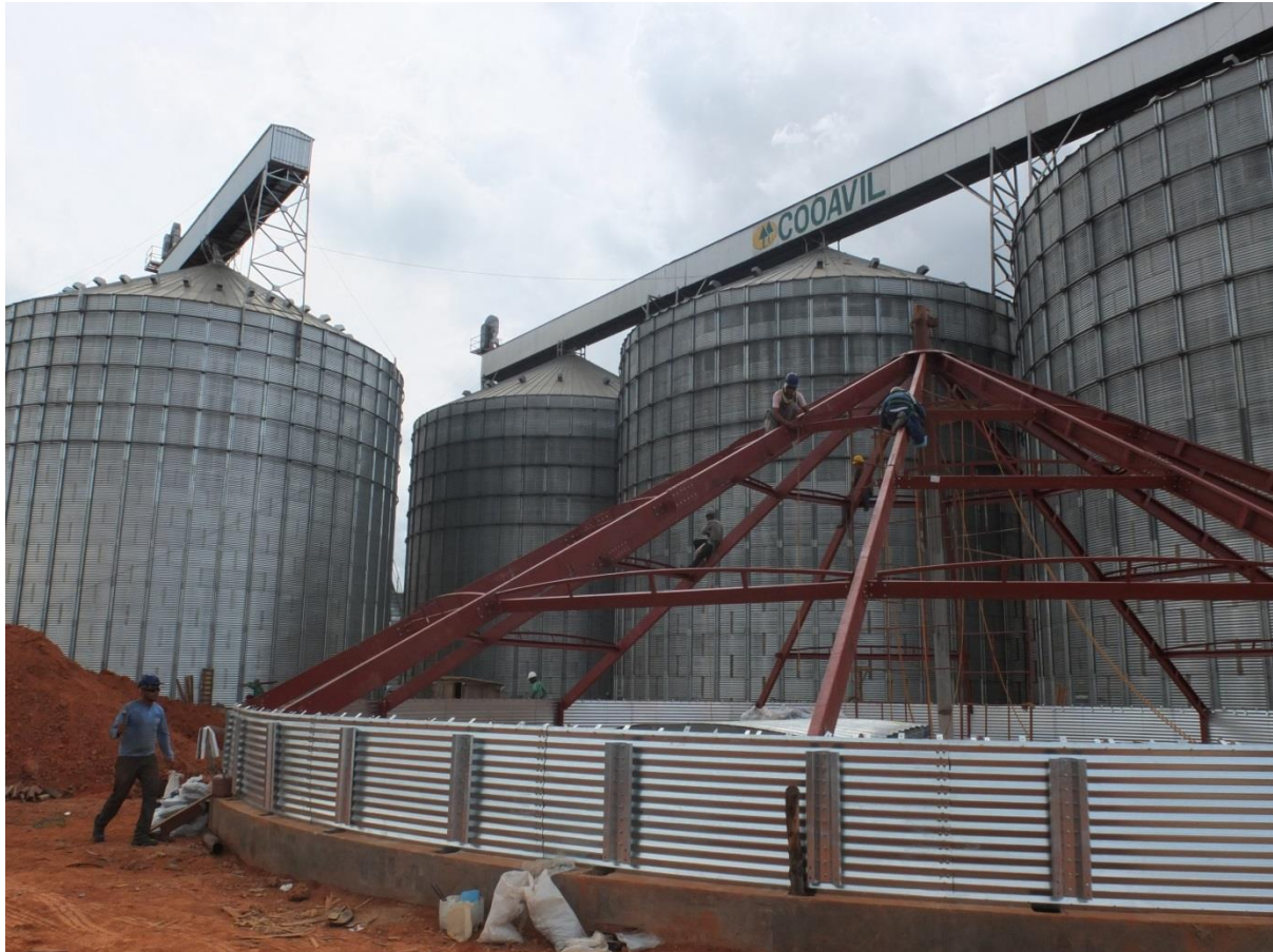
Picture 9 : Coavril building grain silos which will double their storage capacity for the next harvest.
