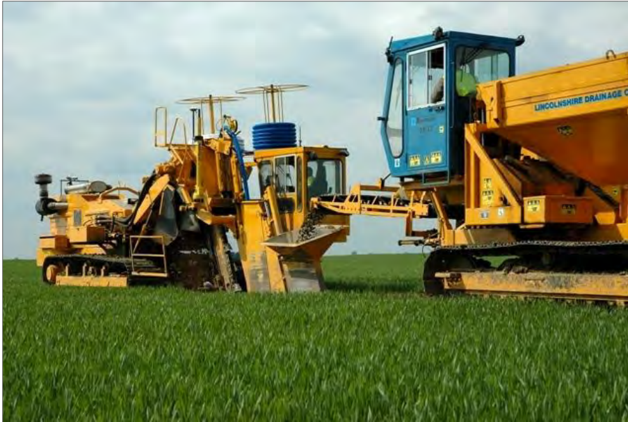
Land Drainage (Source: Mastenbroek 2014)
