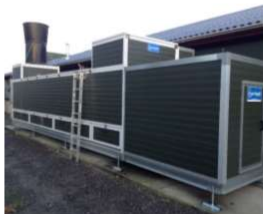
Outside view of commercial broiler shed showing heat exchange unit
