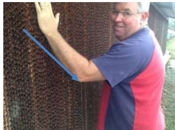
Close up of the cooling pad material and Wayne showing the constant flow of water – dripping from his elbow
