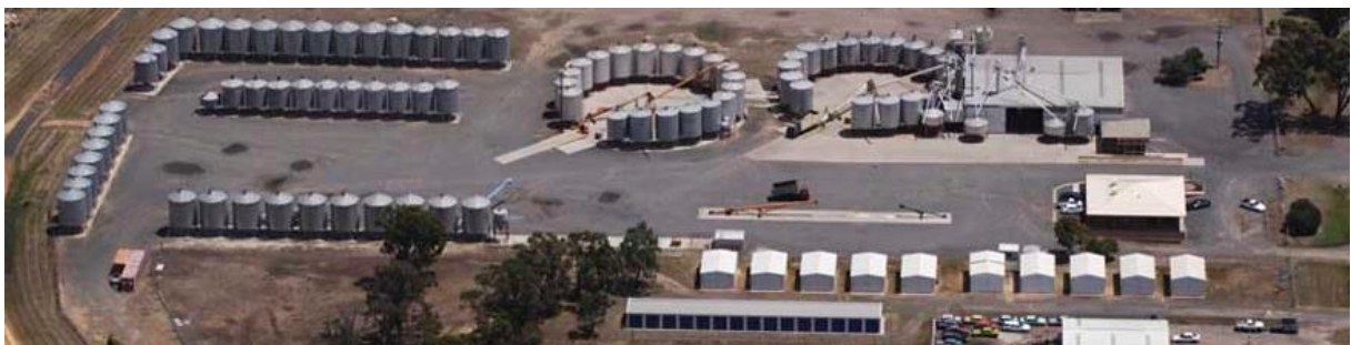
Figure 3: Australia Milling Group processing facility Horsham Victoria.
