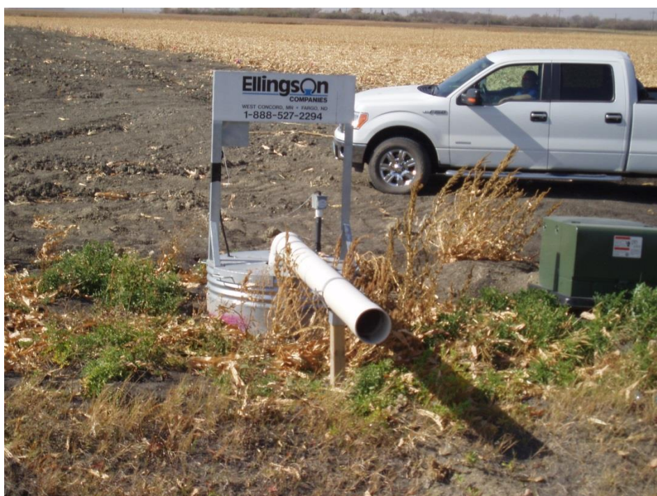
11. Pumped drainage outlet in the Red River Valley, ND, USA
