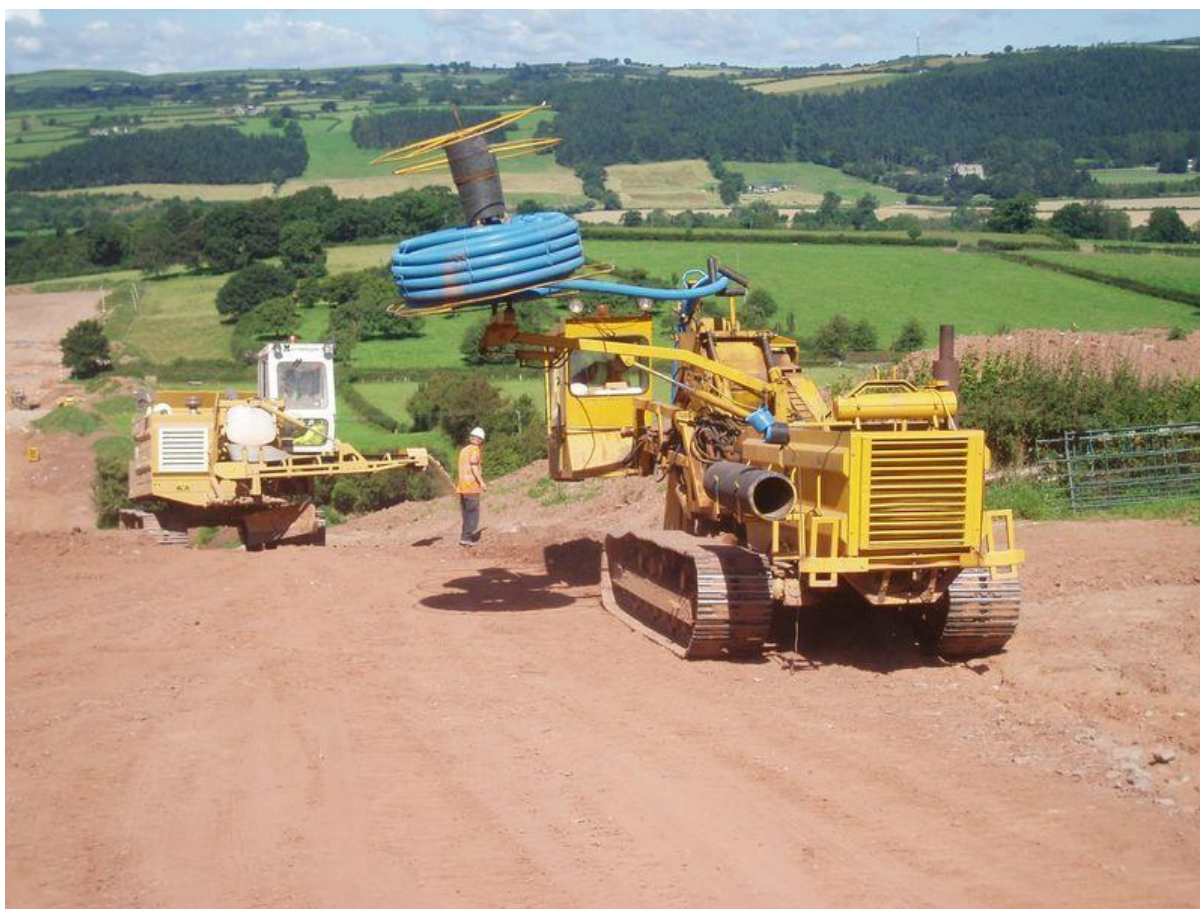
2. Land drainage machine installing pipe
