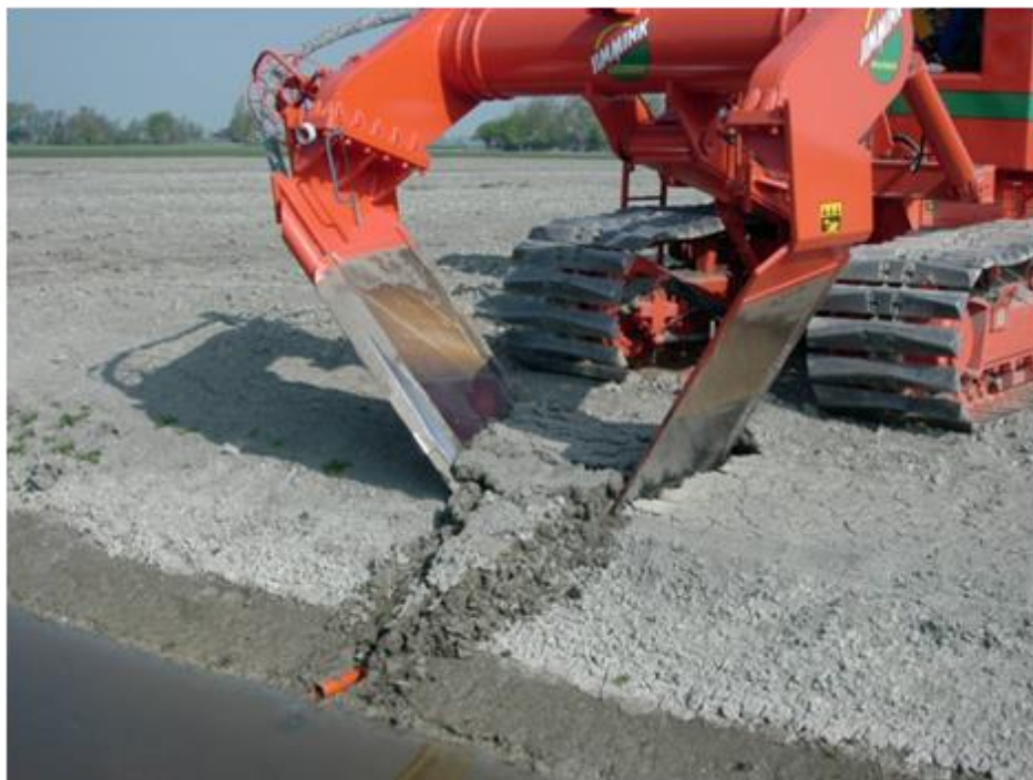
7. Dutch V-plough drainage machine installing pipe – Mastenbroek owned and operated by Jimmick Drainage, The Netherlands
