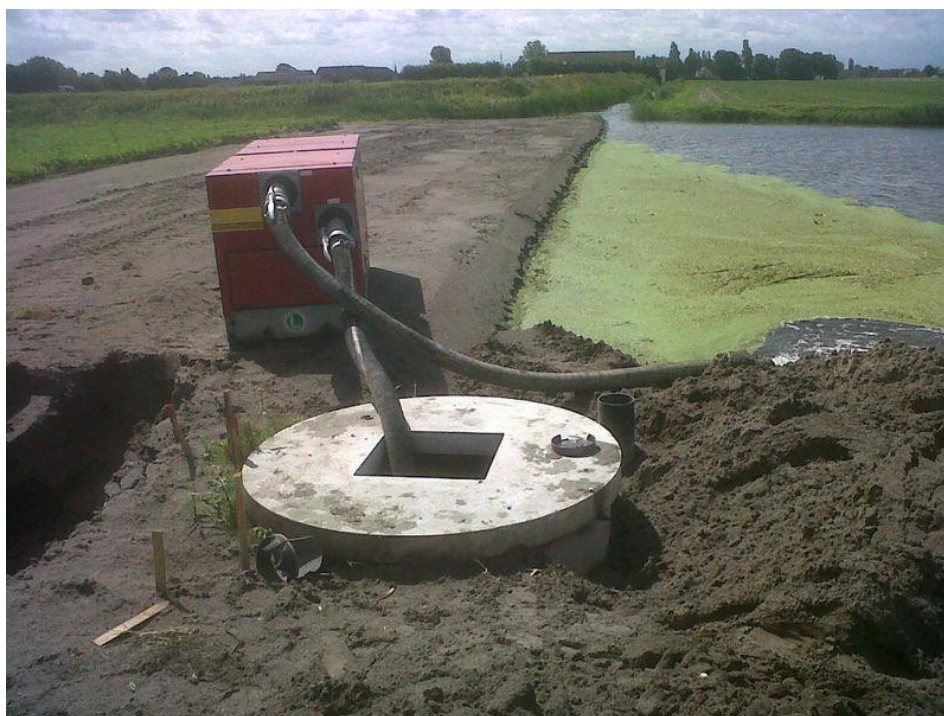
5. Pumping chamber in construction for enclosed drainage scheme, The Netherlands
