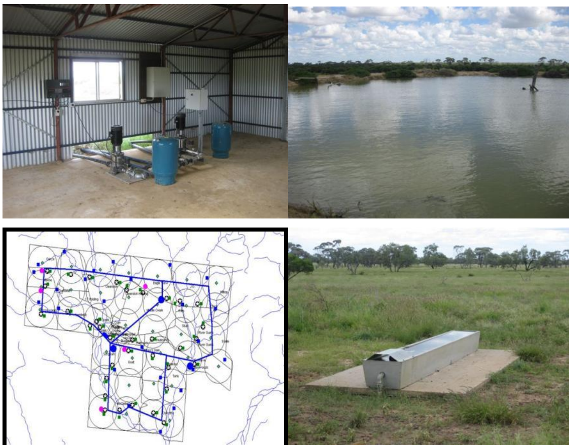
Figure 1 Water Infrastructure at Wakefield Station, Isisford
