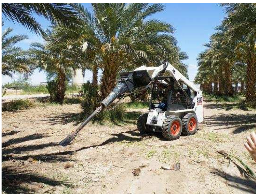
Figure 16: Jackhammer chisel attachment on bobcat ready for offshoot removal Yuma, Arizona 2012
