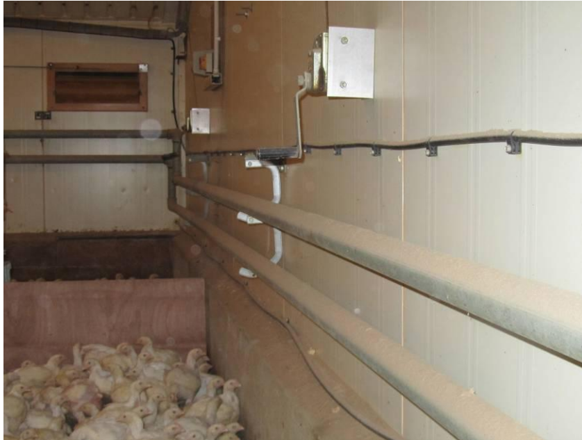
Radiator pipes run around the room to heat the building.
