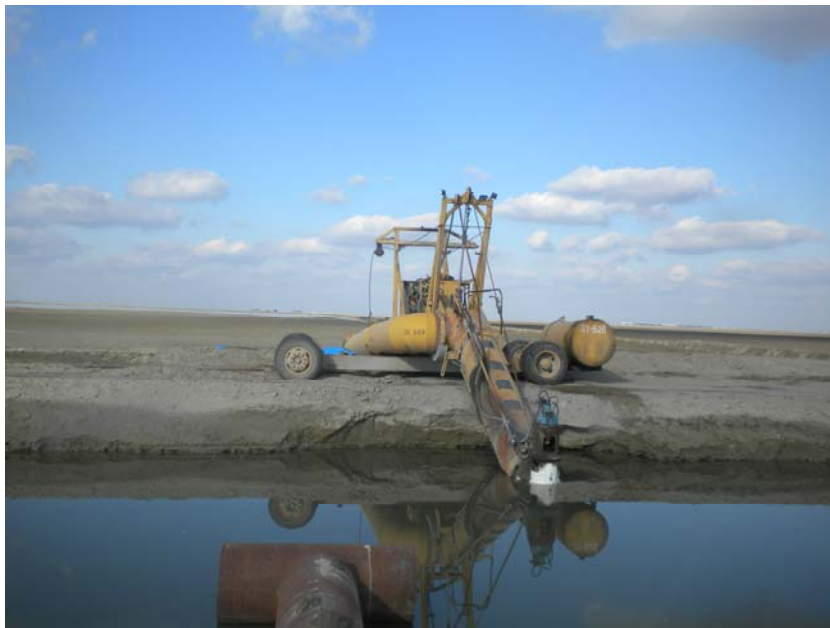
Fig 6: A pump by a dyke at J G Boswells just after it has begun flooding a quarter of a square mile of bare land in preparation for sowing
