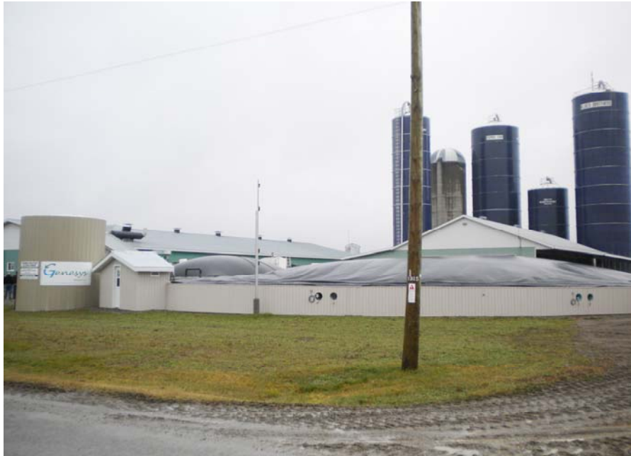
Fig 3: The cow shed and food waste towers in the background with the gas bubble half inflated in the foreground.
