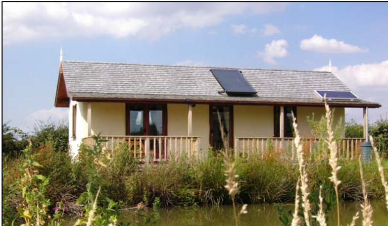
The Straw Bale Cabin - our first straw bale building completed in March 2007. At only 10m by 4m and built on a caravan chassis, this was an ideal starting point for us. The resulting one bedroom "mobile" straw bale holiday home is performing well – and proving a popular tourist destination on our East Yorkshire farm.
