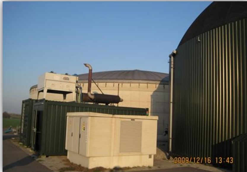
HOST AD, Holland, Plant showing Electrical Compound, Control Room, First Stage Digester and Digestate Storage
