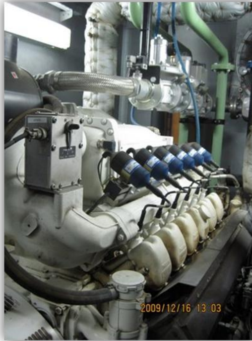
Gas engine running on Biogas generating electricity (Man Rollo)
