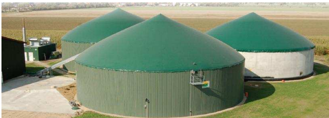
Figure 4: Digester at Lowbrook Farm. Source: Farming Futures
