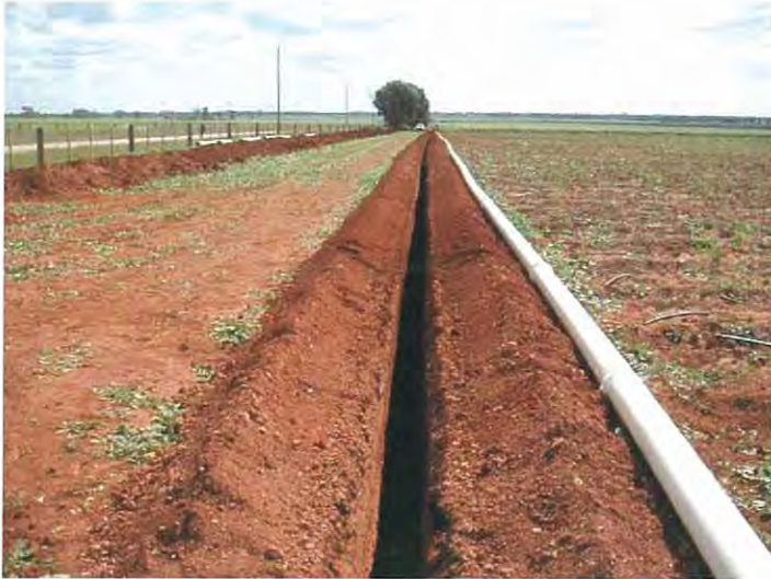
SDI being installed for a processing tomato crop
