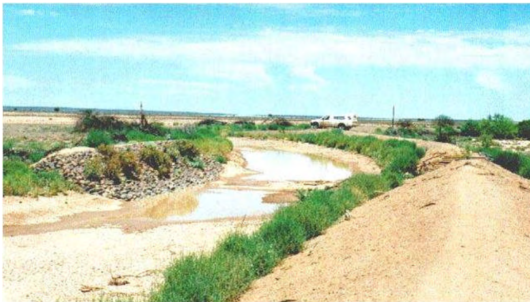
#38 Cement weir in the Karoo Region, South Africa. Side view showing channel for dispersing water across the flats. Photo c/o Mr. Charl du Plessis, Western Cape Dept of Agriculture
