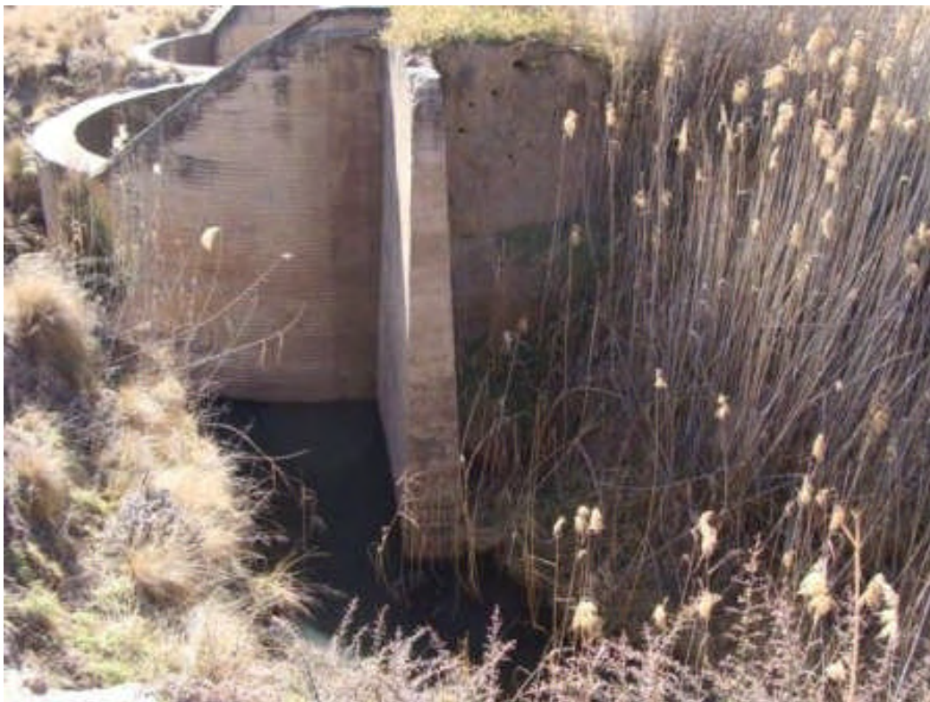
#09 Cement weir near Ladybrand, Free State, South Africa. The walls were not keyed into the landscape far enough and have failed. A total waste of resources due to poor design and lack of maintenance.
