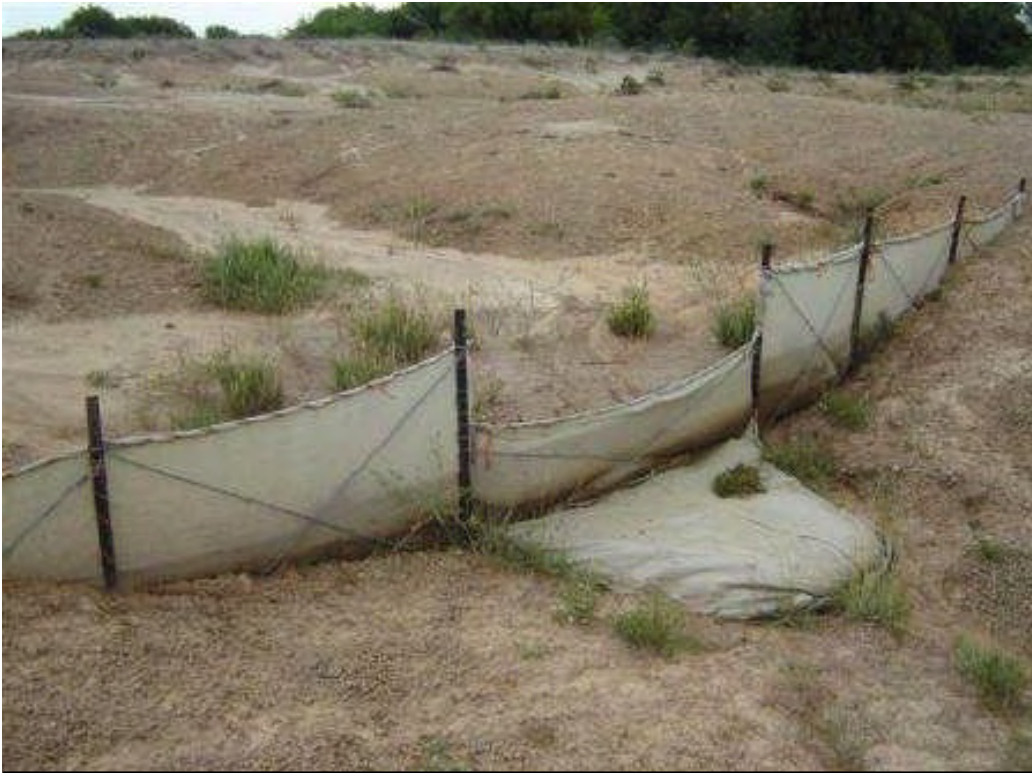
#51 Using star pickets and synthetic cloth to form a temporary “silt fence”. Photo c/o Mr. Chris Smith, Free State Department of Agriculture.
