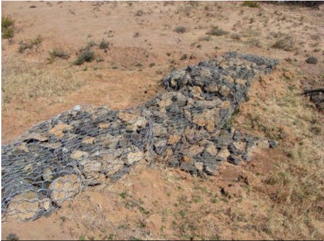
#47 A small gabion structure trial by the Free State Department of Agriculture, near Ladybrand, Free State, South Africa.
