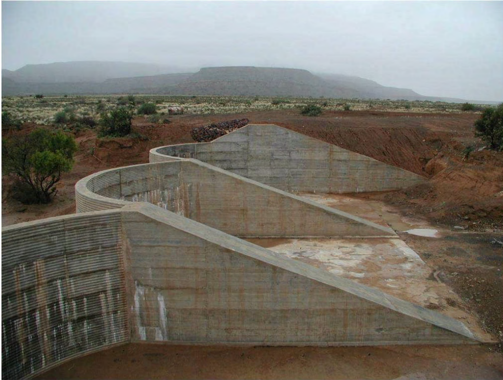
#35 New cement weir in the Karoo Region, South Africa. Water flows from left to right over the low point in an earth wall. Photo c/o Mr. Charl du Plessis, Western Cape Dept of Agriculture, Elsenburg, Western Cape, South Africa.
