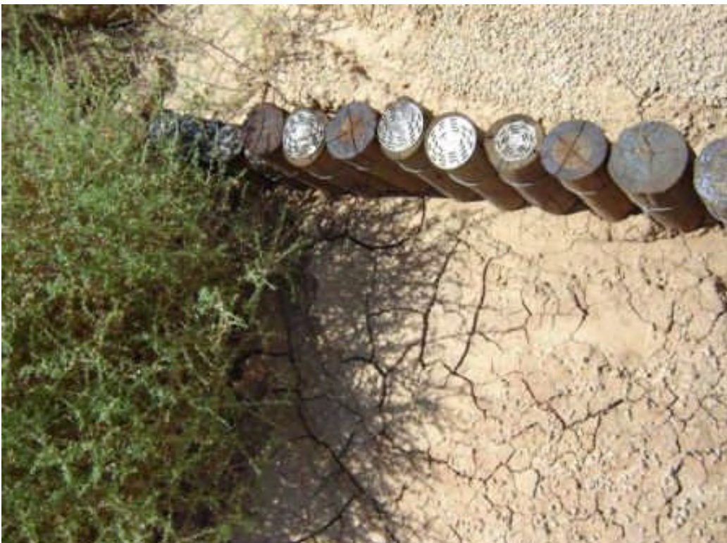
#52 Using pine bollards twitched together to form a “silt fence”. Photo c/o Mr. Chris Smith, Free State Department of Agriculture.
