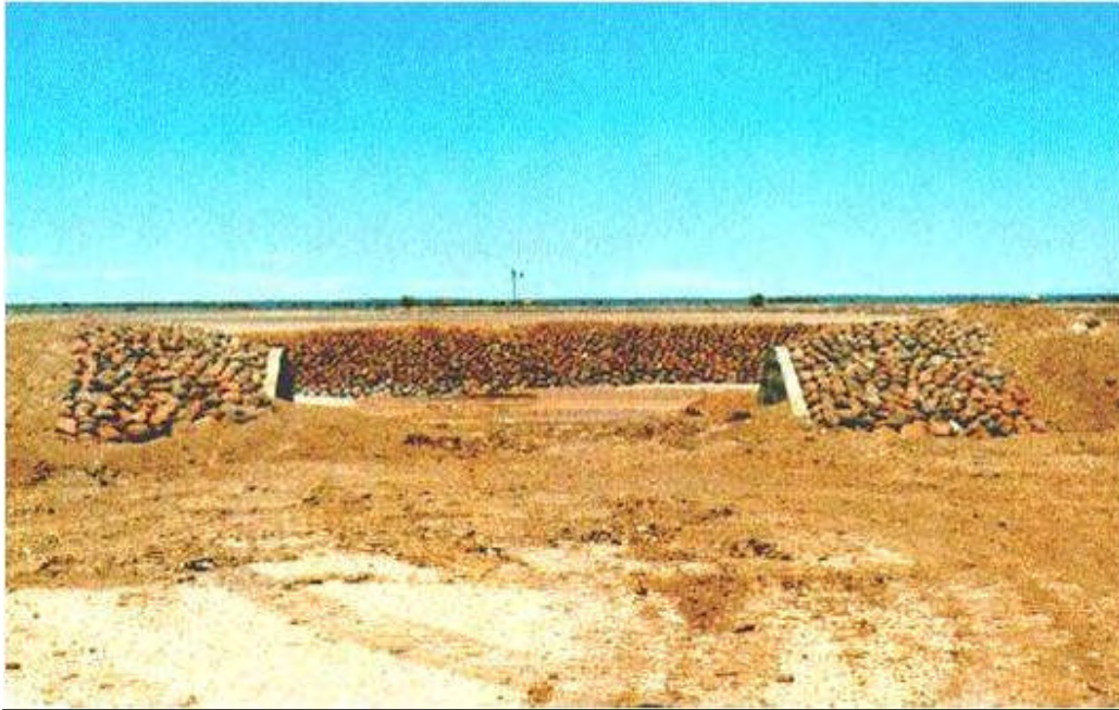
#37 Stone Gabion and Cement weir in the Karoo Region, South Africa. Note Gabion wall in downstream area to diffuse the concentrated water flow. Photo c/o Mr. Charl du Plessis, Western Cape Dept of Agriculture
