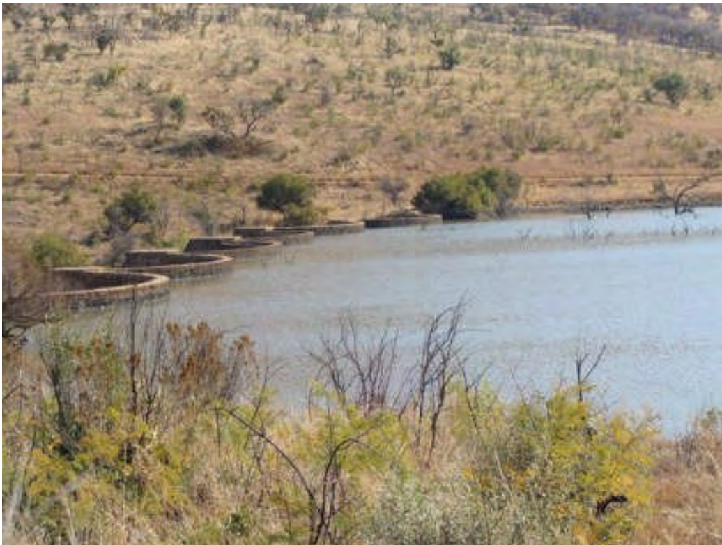
#34 Cement weir in the Pilanesberg National Park, South Africa. Note half moon design of wall for added strength for minimal concrete.
