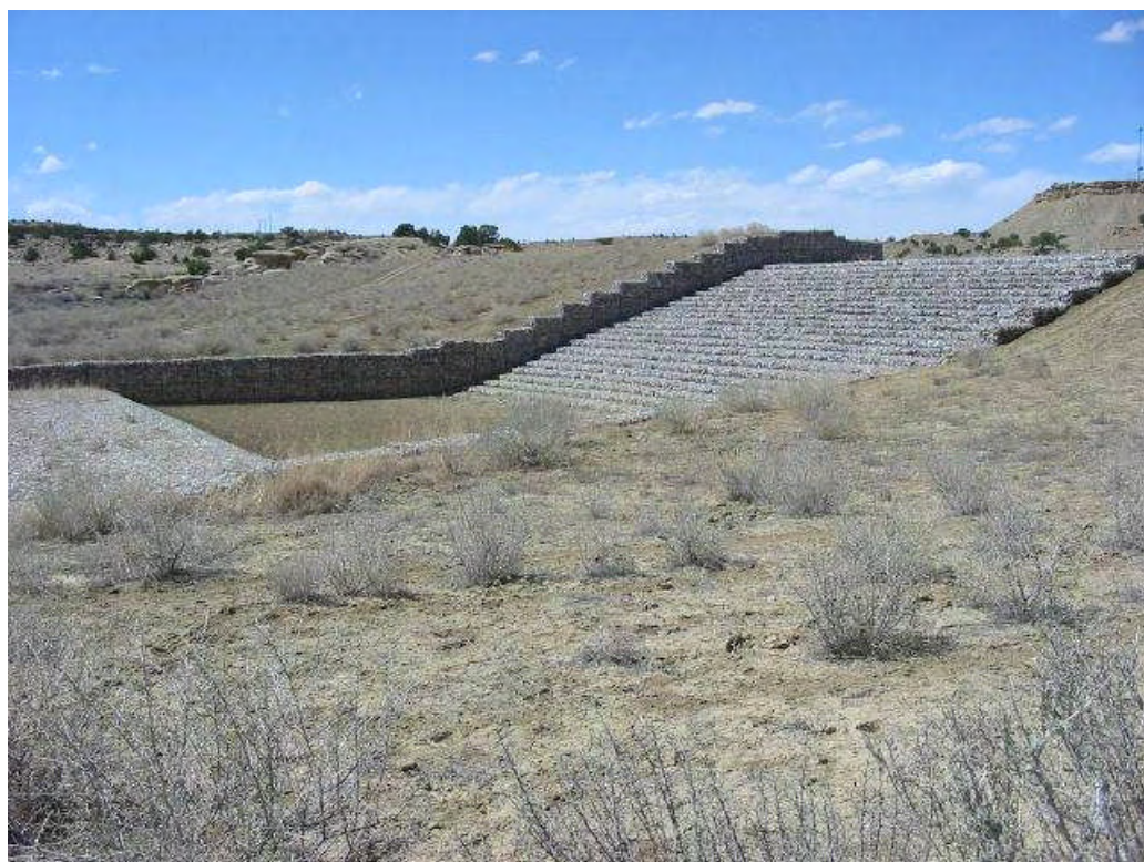
#54 An extensive stepped Gabion structure, New Mexico. Photo c/o Mr. Steve Fischer, BLM, Albuquerque, New Mexico.
