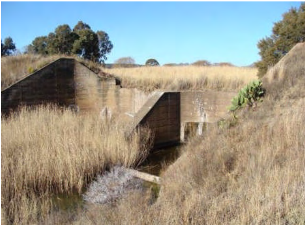
#08 Cement weir on Sparta Farm, the upstream side has completely filled with soil and pasture. A fantastic example of appropriate engineering.
