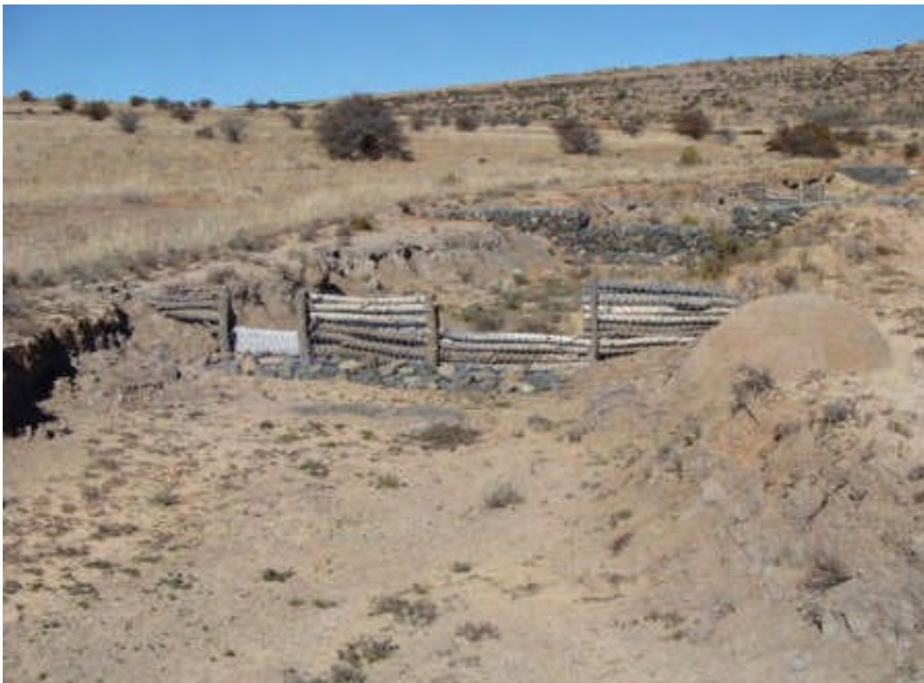
#50 Various trials of erosion control structures by the Free State Department of Agriculture, near Ladybrand, Free State, South Africa.
