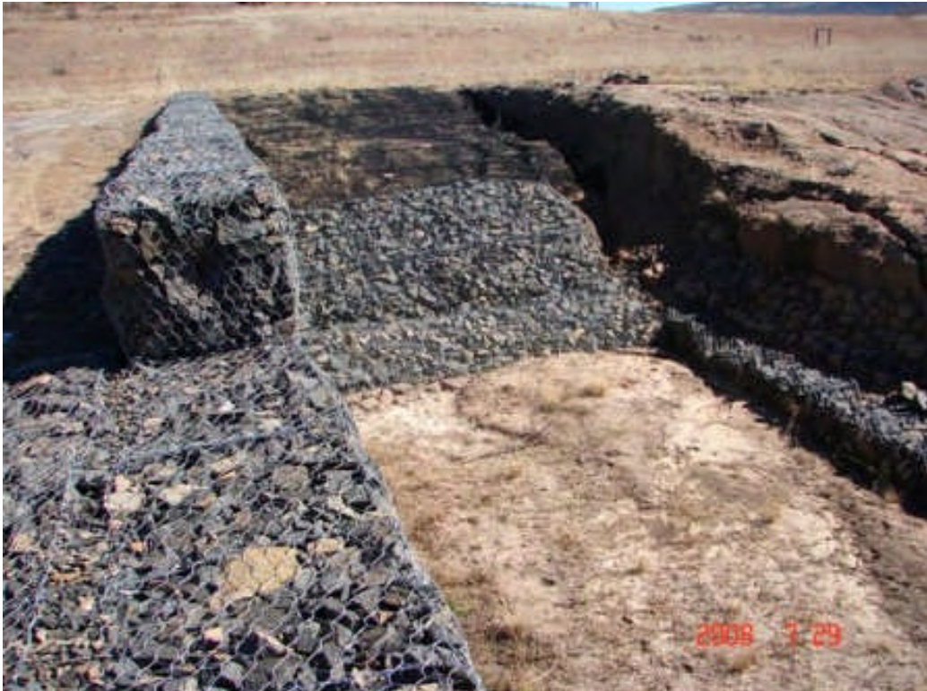
#43 Gabion splash zone pool to dampen the energy of the falling water, near Ladybrand, Free State, South Africa. Photo c/o Prof Klaus Kellner.
