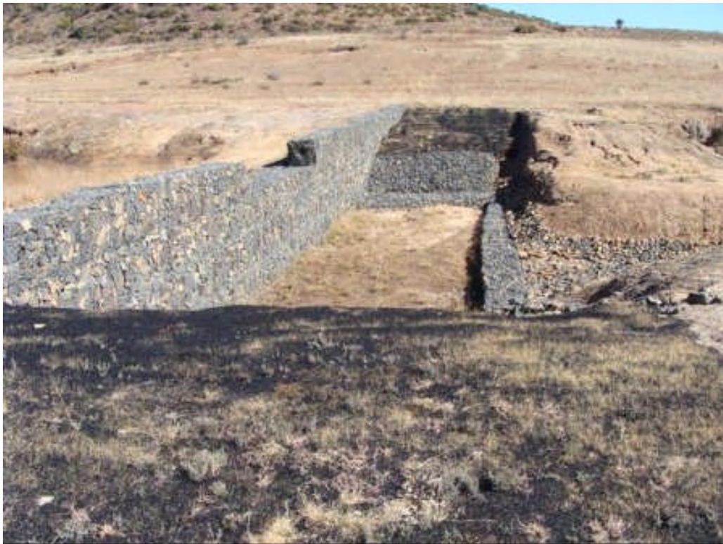
#41 Major gabion structure trial, by the Free State Department of Agriculture, near Ladybrand, Free State, South Africa.
