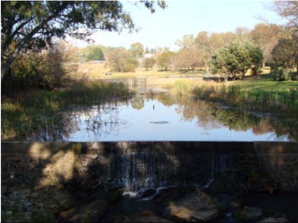
#31 Cement weir in the ForeverSA Resort, Badplaas, Mpumalanga, South Africa. Second structure in background. Very effective design onto rock spillway.
