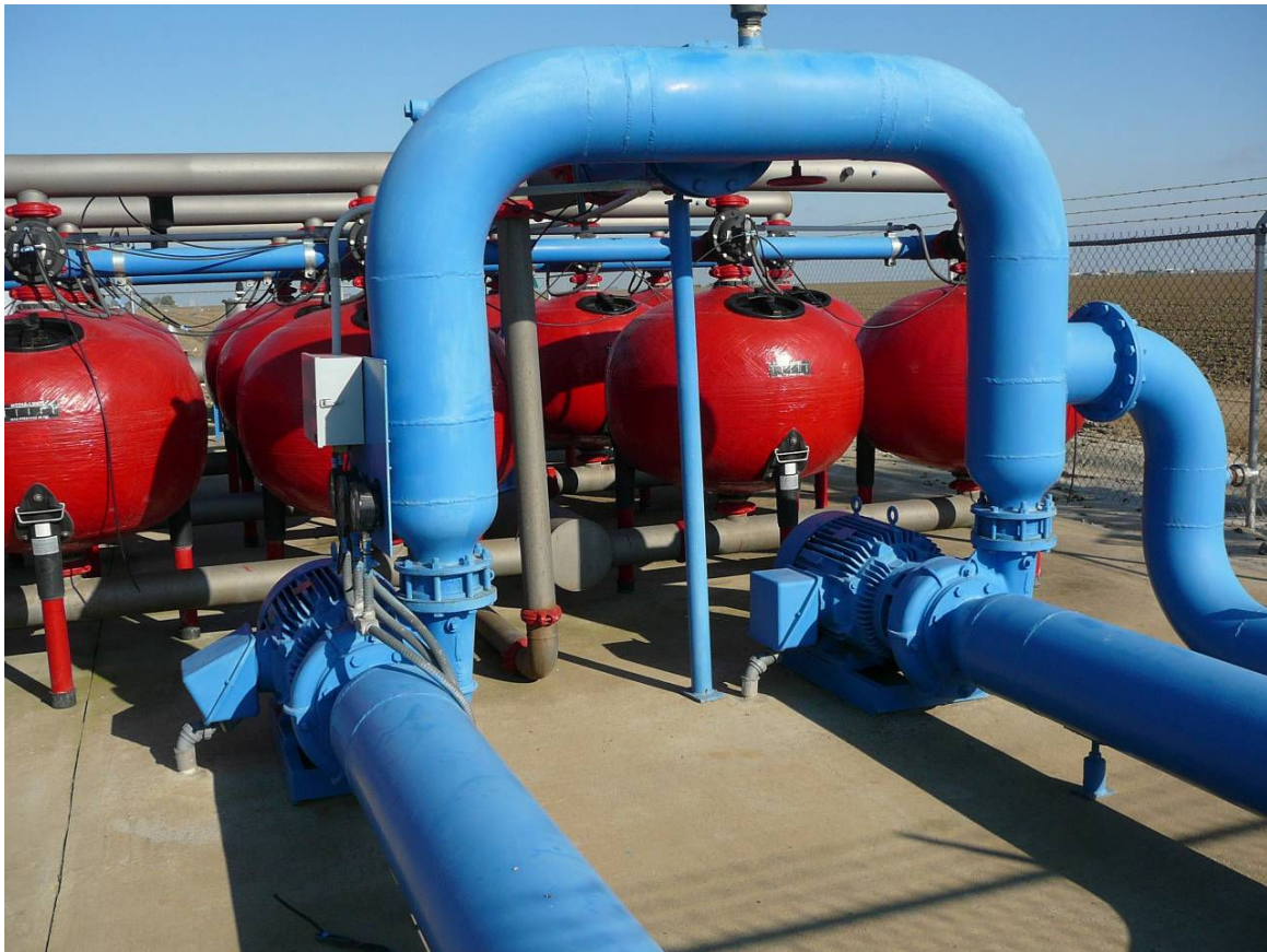
Sand filters play an important role in the filtering of irrigation water. Sub surface pipe had been in place for 8 years at this property.
