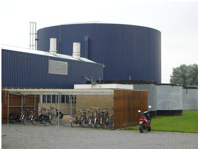
Picture 2. Large, vertical heat storage or buffer tank. The Netherlands.
