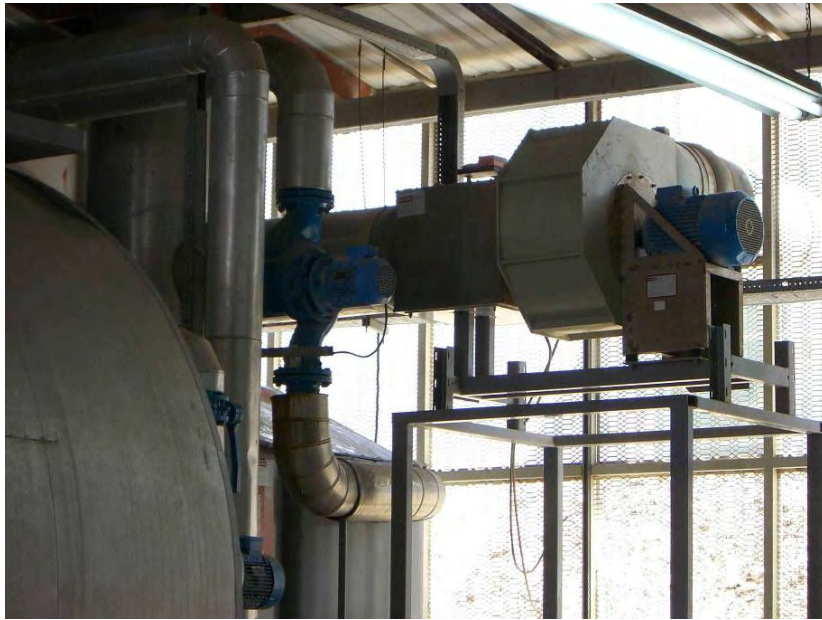
Picture 1. Carbon dioxide extraction fan. Mexico.
