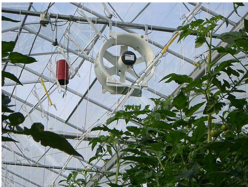
Picture 7. Glasshouse venting panel. Note stirring fan. The Netherlands.
