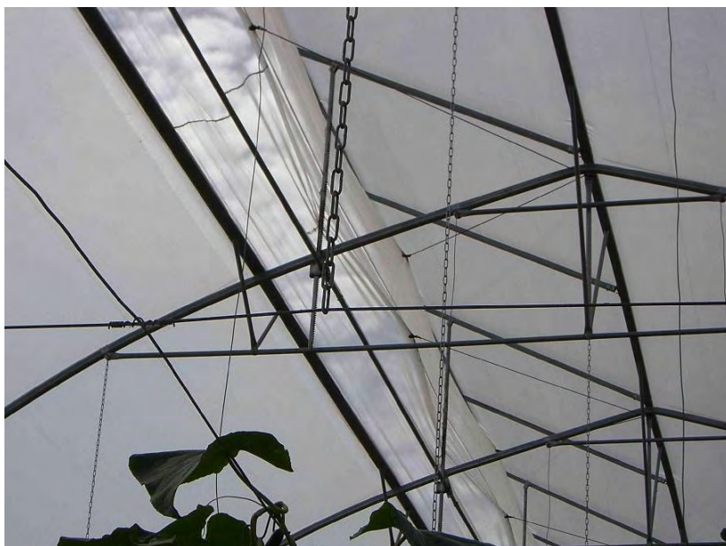
Picture 6. Continuous vent in plastic greenhouse. Note insect screen. Mexico.
