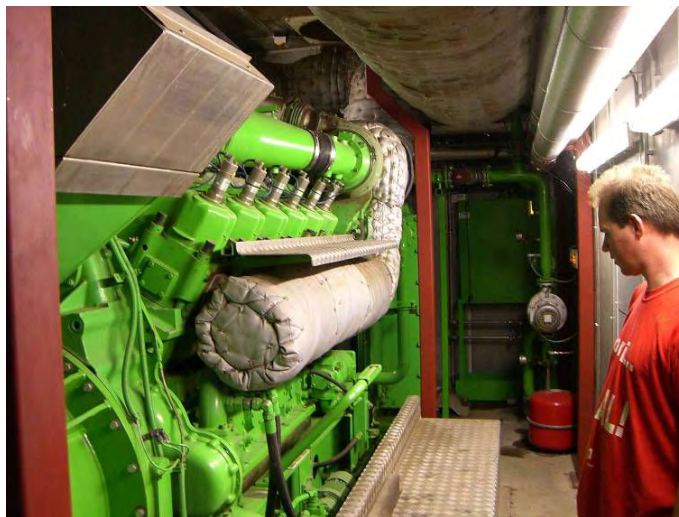
Picture 5. Co-generation unit. Generator. The Netherlands.
