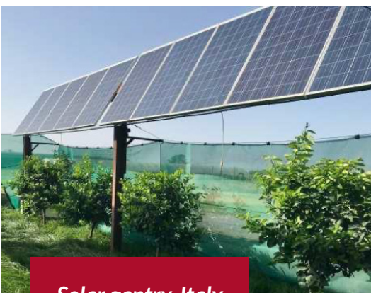
Solar gantry, Italy
