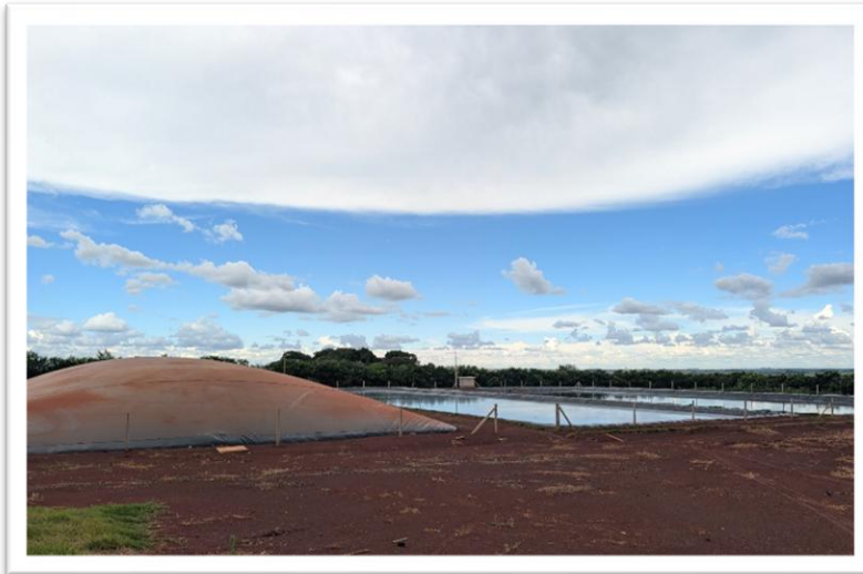
Figure 15: Methane capture over pig slurry pits,
