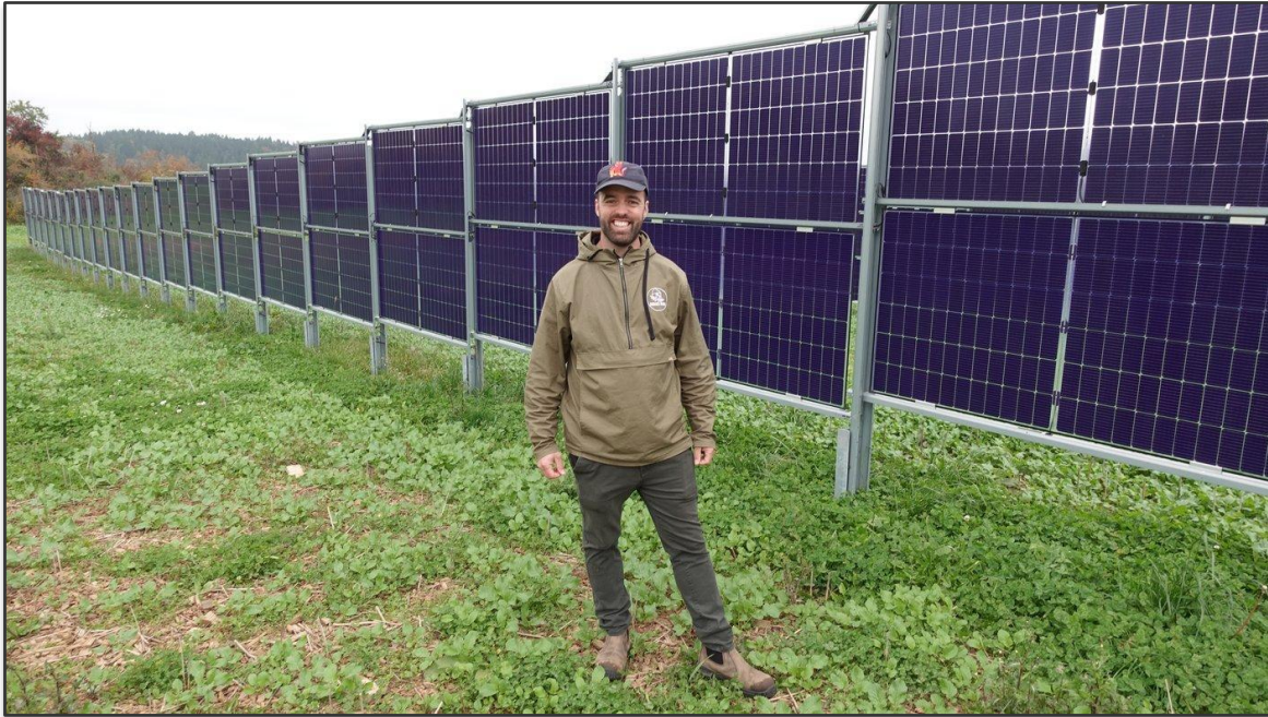
Figure 11: Vertical bifacial agrivoltaic panels on a working farm, southern Germany, energy generation and active crop production from the same land. Full machinery access maintained beneath.
