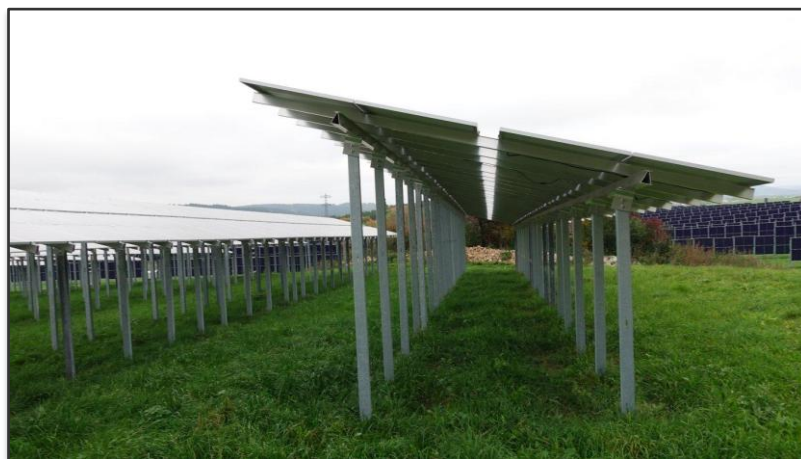
Figure 13: Elevated agrivoltaic panels on a working farm, southern Germany. Panels raised high enough for cattle to graze beneath and small machinery to pass. Simple design, genuine dual use.
