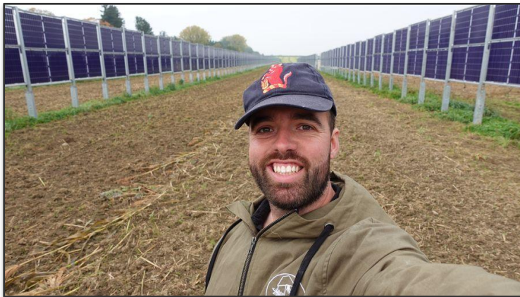
Figure 14: Between the rows of a vertical agrivoltaic system, Germany. Tillage running right to the base of the panels. No wasted ground, no buffer zone. Farming and energy generation sharing the same soil.
