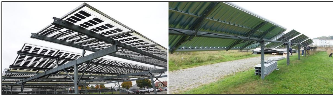
Figure 12: Southern Germany agrivoltaics demonstration site. Left: transparent PV panels allowing light through to crops beneath. Right: tilting panels that track the sun, outperforming fixed arrays by up to 15 per cent while folding clear for machinery.
