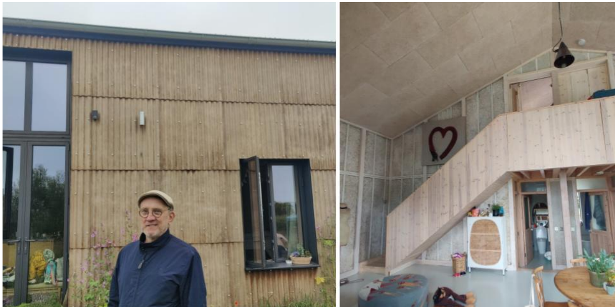
Figure 6.3 Steve Barron at Margent Farm, Cambridgeshire - a home made out of hempcrete, hemp plaster and corrugated hemp fibre composite panels grown on the farm.
