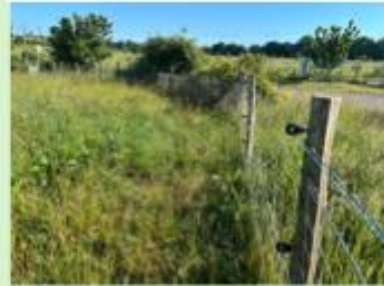
Gold standard boundary fencing: solid fence with electric
