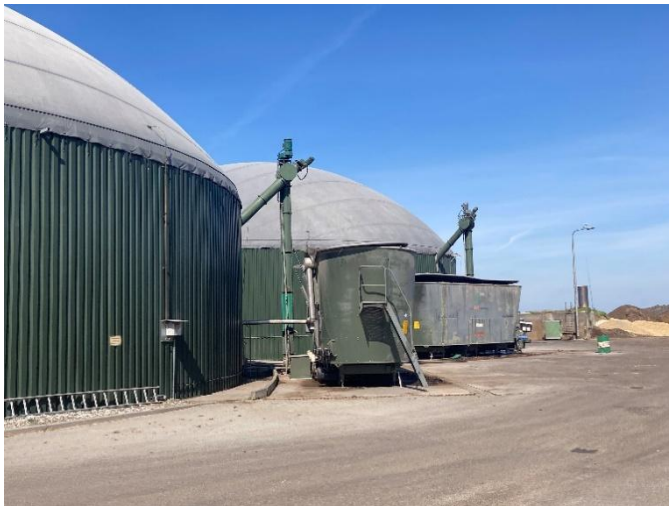
Figure 8. Anaerobic Digester Plant. Source: Author's own.
