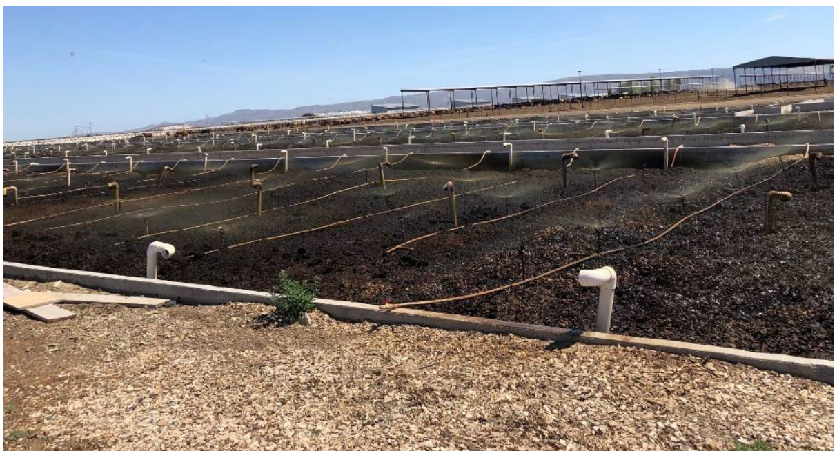
Liquid from the flume wash being pumped onto the Biofiltro BIDA at Royal Dairy.
