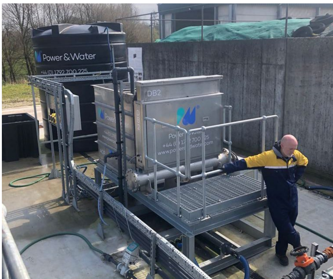
The “Soneco” electrode, marked DB2 on the front of the AOP “Advanced Oxidation Process” tank.
