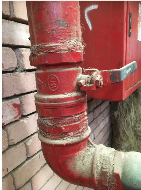
Figure 11. Flax fibre used in plumbing at Motaz Elkholy warehouse in Egypt
