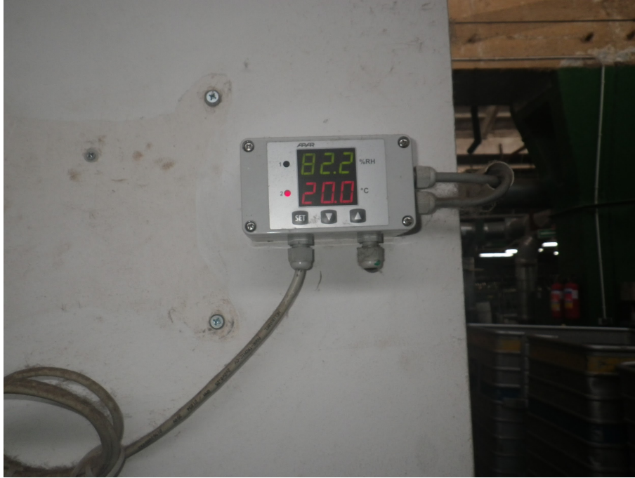
Figure 7: A humidity and temperature monitoring device, picture taken at the Safilin Mill in Poland
