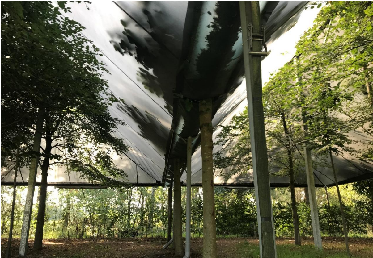
Figure 107: Looking up at the roof of the tree/fabric hybrid structure. Author's own photo.
