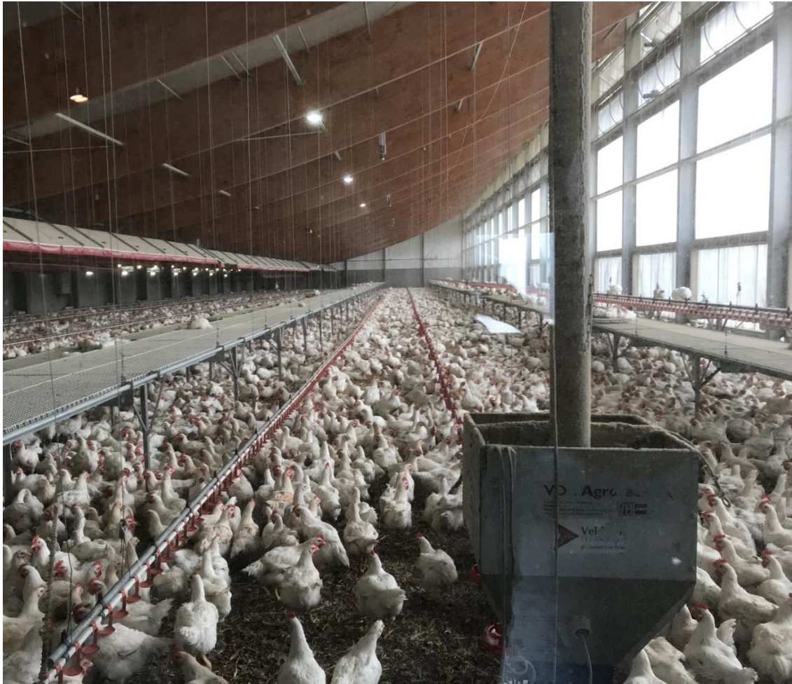
Figure 51: Interior of Windstreek House, with translucent northern wall and timber roof trusses. Author's own photo.
