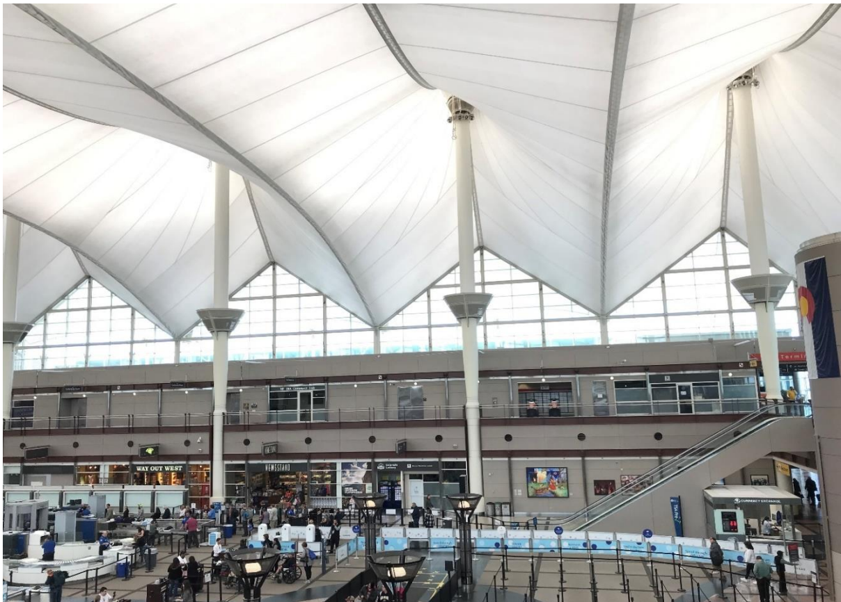
Figure 104: Tensegrity roof structure with tensile fabric covering at Denver Airport's main terminal. Author's own photo.
