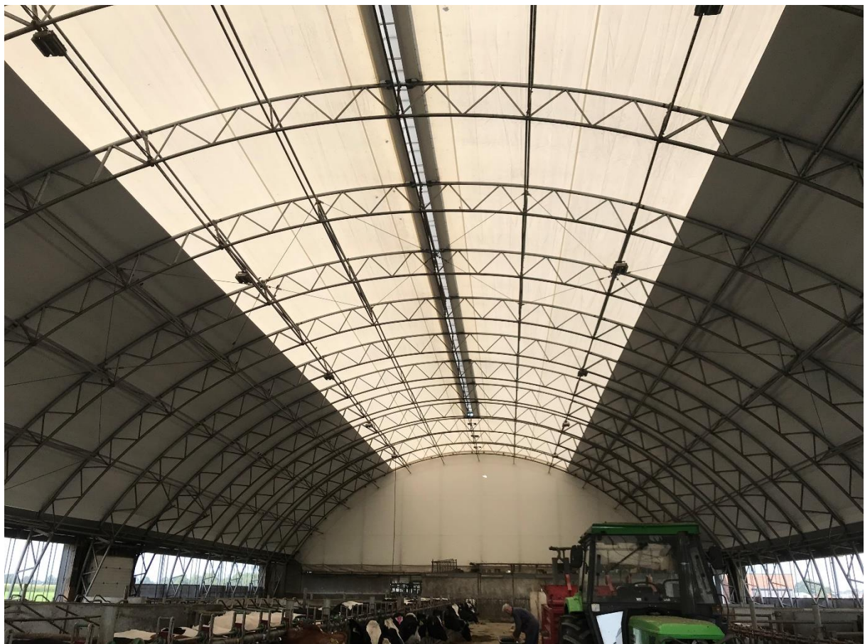
Figure 48: Looking up at the roof structure and different fabric types. Author's own photo.
