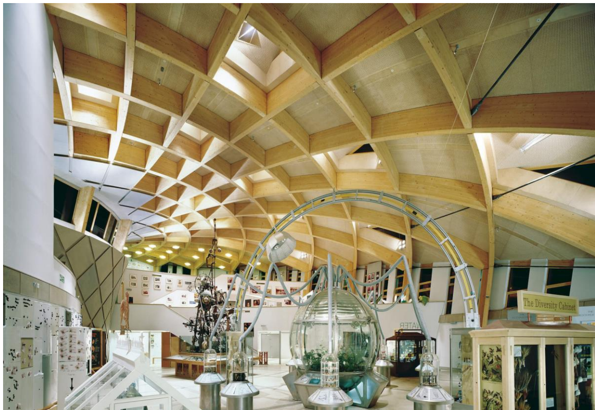
Figure 13: Interior of the Core building, showing laminated timber sectional roof. Photo from Grimshaw Architects.
