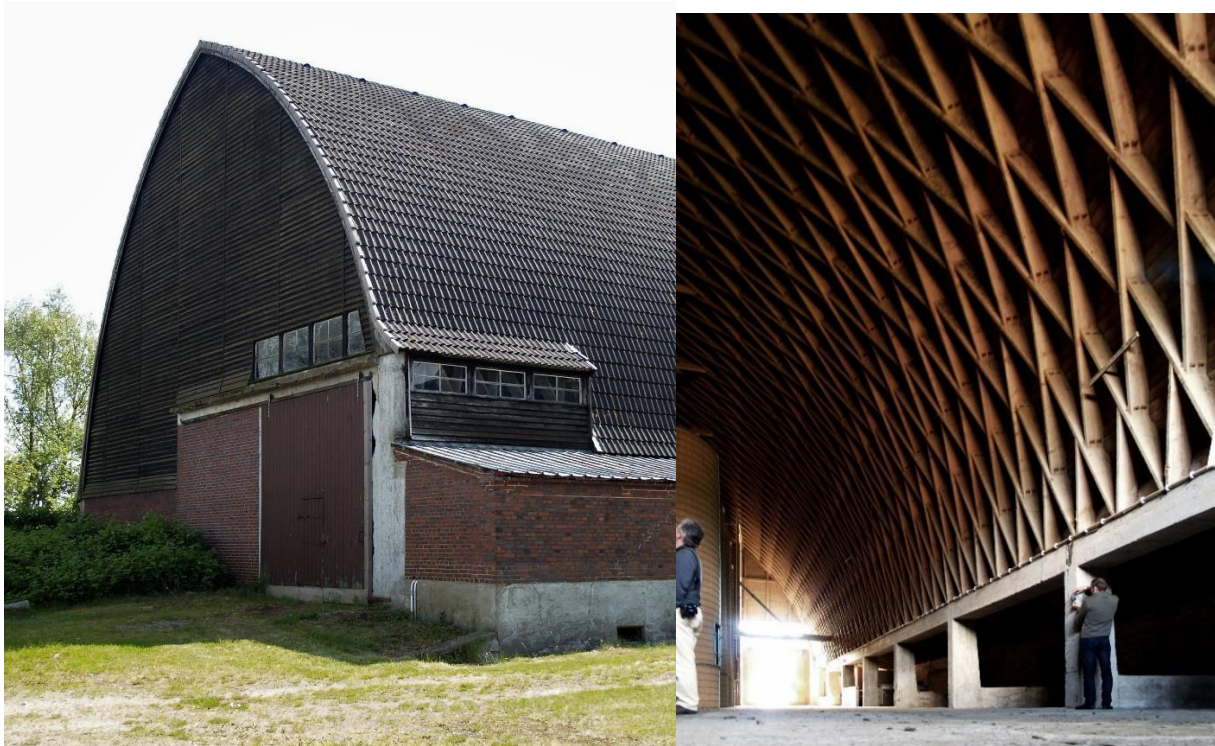
Figure 101: Gut Garkau farm building by Hugo Haring, Germany, featuring a lamella roof. Photos: Seier & Seier.
