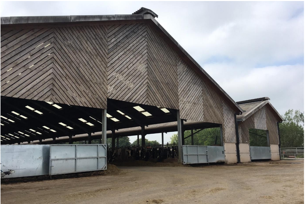
Figure 27: Exterior of a modern dairy barn, Cheshire. Note the angled layout of boarding to reduce timber wastage. Photo from The Barnston Estate.
