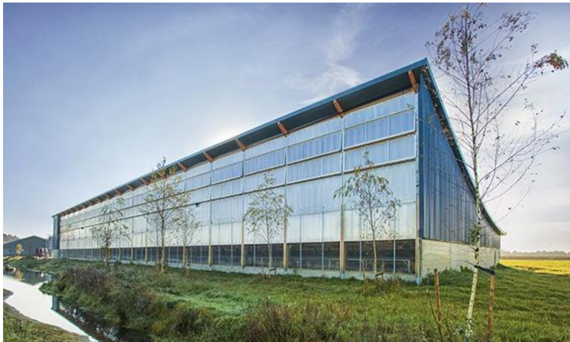
Figure 52: The northern wall of Windstreek House, with polycarbonate wall for maximum natural light. Photo: VDL Agrotech.
