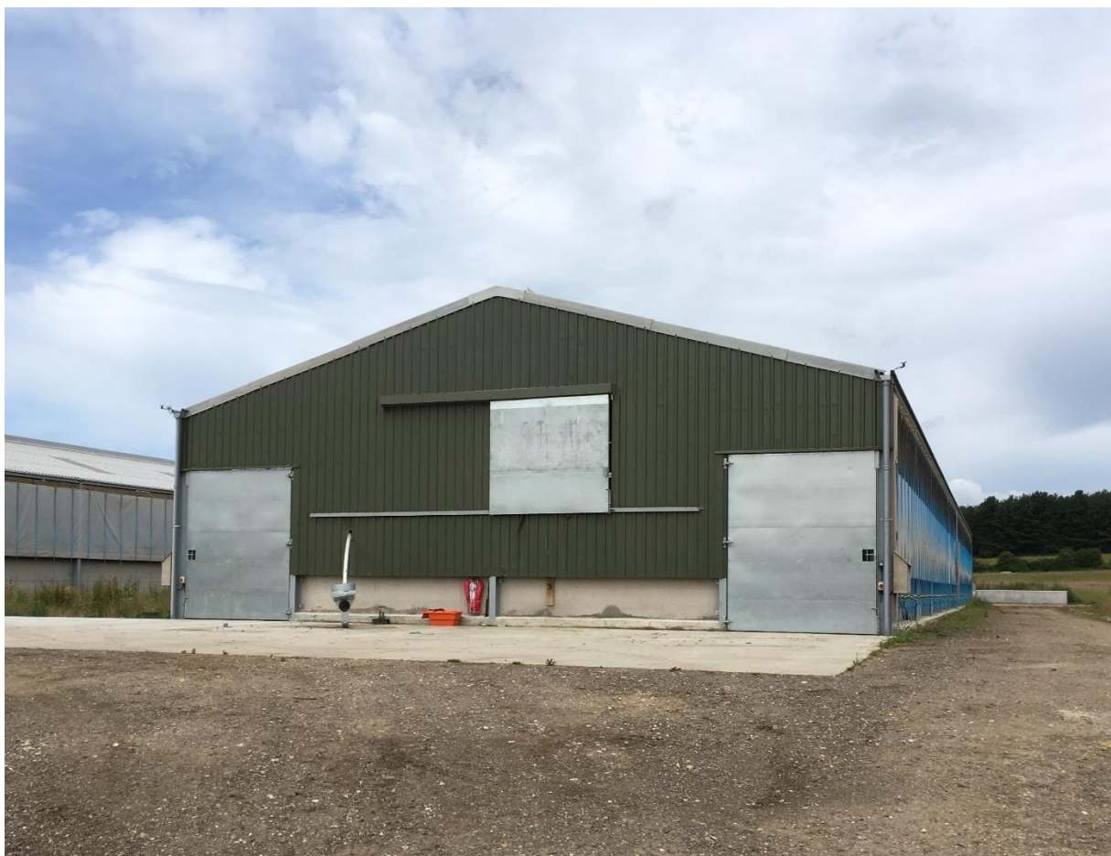
Figure 29: External photo of a modern straw bedded pig shed, with automated side curtains for ventilation and temperature control. Author's own photo.
