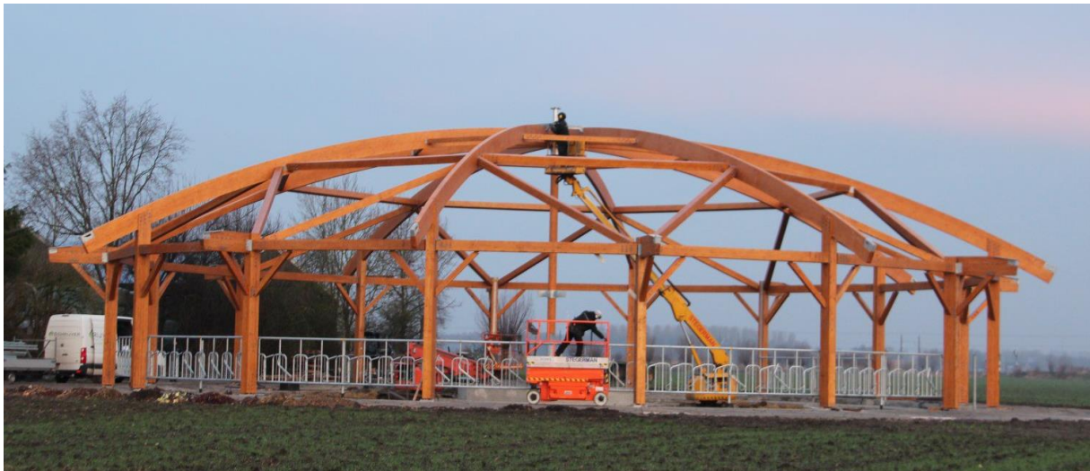
Figure 39: A timber framed roundhouse being constructed, awaiting tensile fabric roofing. Photo: ID Agro.
