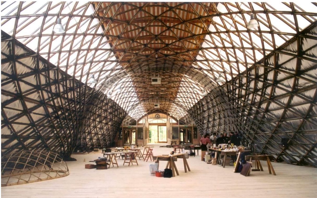
Figure 92: A full size gridshell building at the Weald and Downland Museum, by Edward Cullinan Architects and Buro Happold. Photo: Buro Happold.
