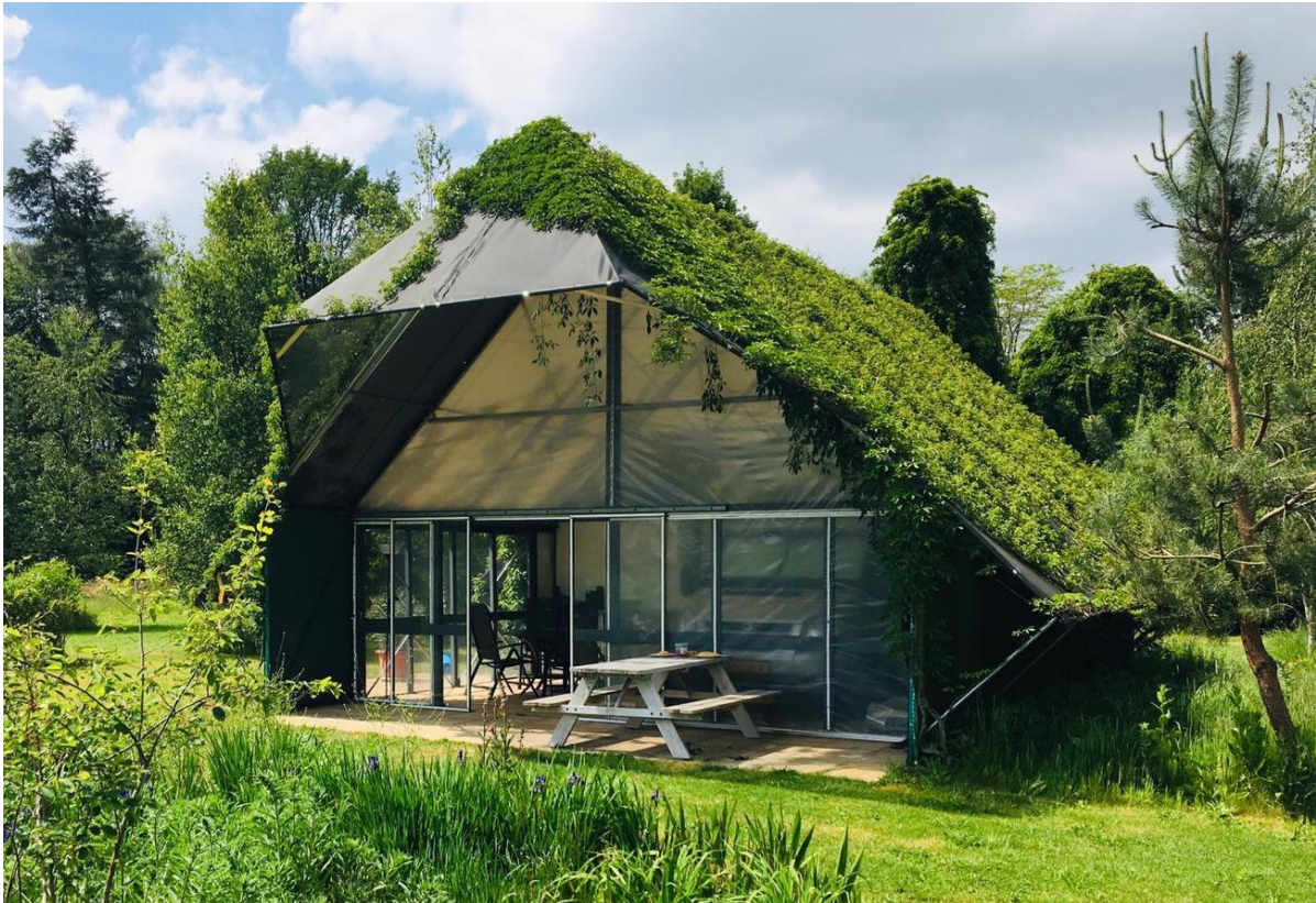
Figure 109: Steel framed structure with tensile fabric roof and plants grown over to provide shade. Photo: Bram Pape.
