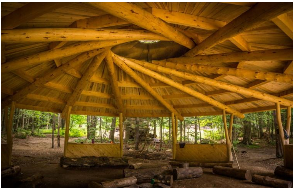
Figure 100: A roundhouse with reciprocal roof structure, self-supporting. Photo: Timber Homes Vermont.
