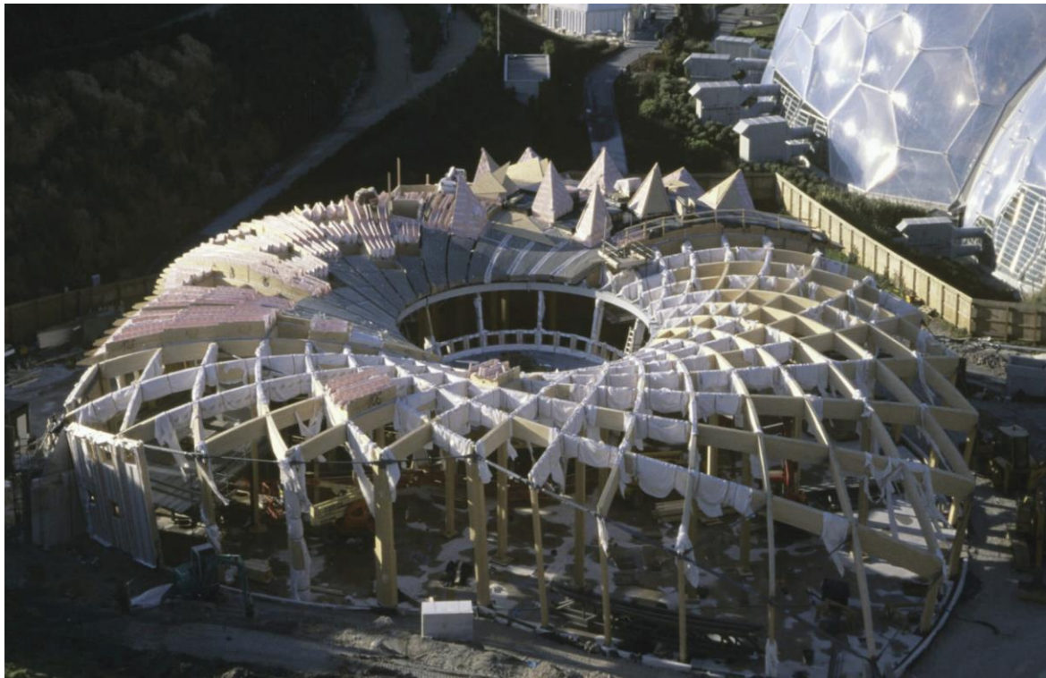
Figure 12: The Core building, Eden Project, during construction. Note the spiral – a “biomorphic” form. Photo by Grimshaw Architects.
