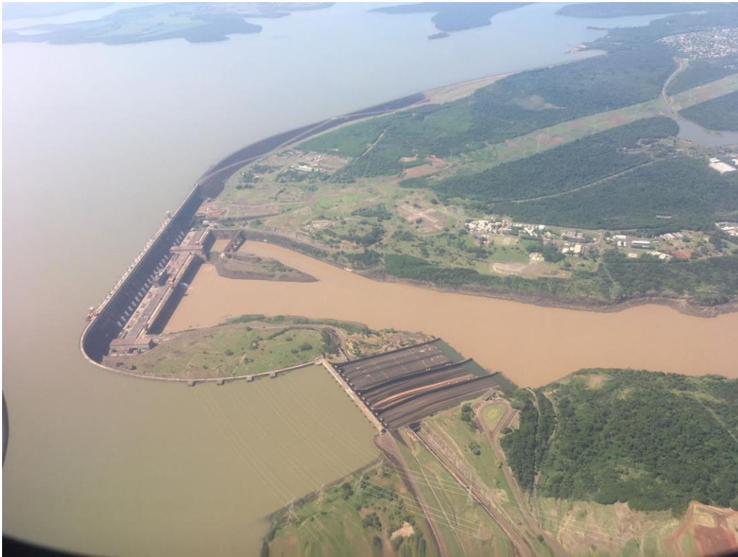
Figure 9: The Itaipu Dam, the largest hydroelectric power supply in the world and one of the seven man-made wonders of the world, Foz do Iguazu, Brazil (Source: Author, 2018)
