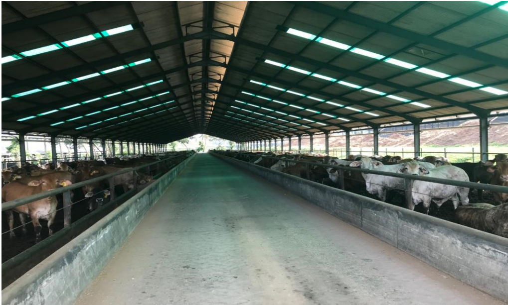
Figure 12: A good example of raised ridge cap housing at JJAA Feedlot, Lampung Indonesia (Source: Author, July 2018)
